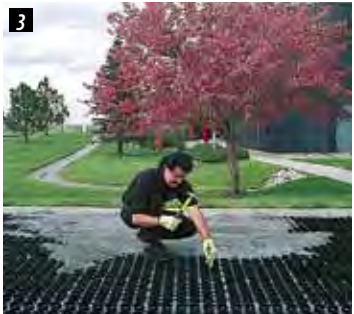
Secure mats with anchors provided (size and type may vary).
