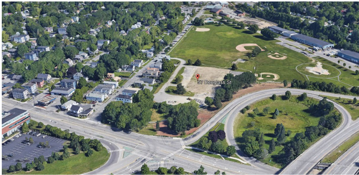
Figure 2: Aerial View of Site (facing north)
