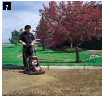
Place and compact sand and gravel base course.
