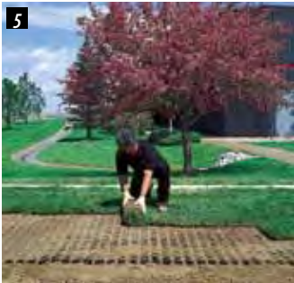
Hydroseed or lay sod.
