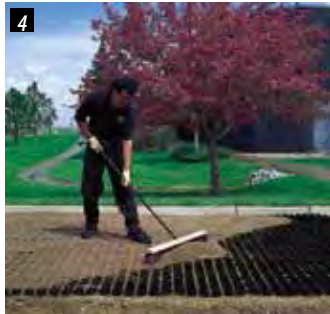
Fill rings with clean sharp concrete sand.
