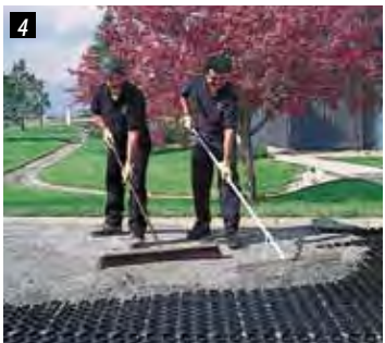
Fill rings with clean gravel.
