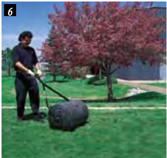
Roll sod with heavy roller.
