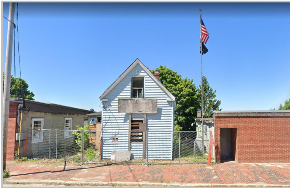
Figure 2: Existing Condition of 180 Washington Avenue
