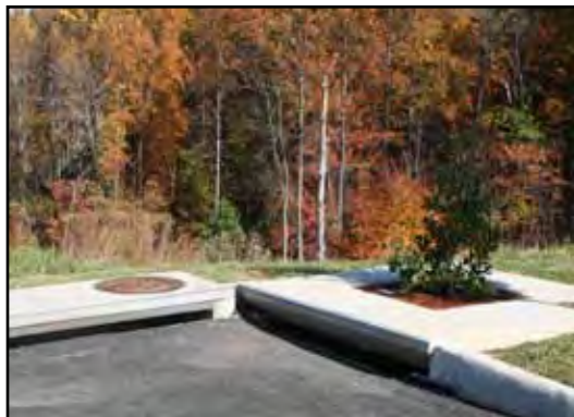
1. Inspection of Filterra and surrounding area
