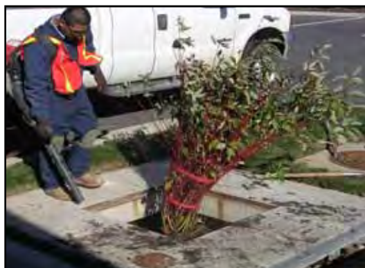
5. Clean area around Filterra
