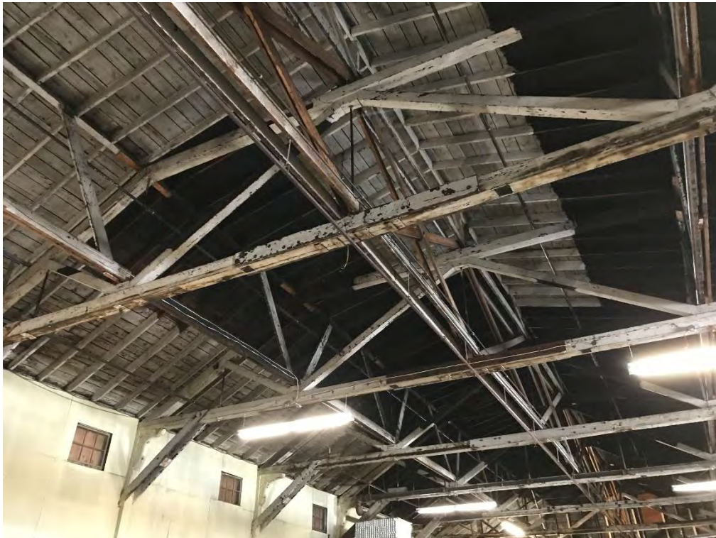
Photo 20. Warehouse No. 4. High bay wood roof trusses.
