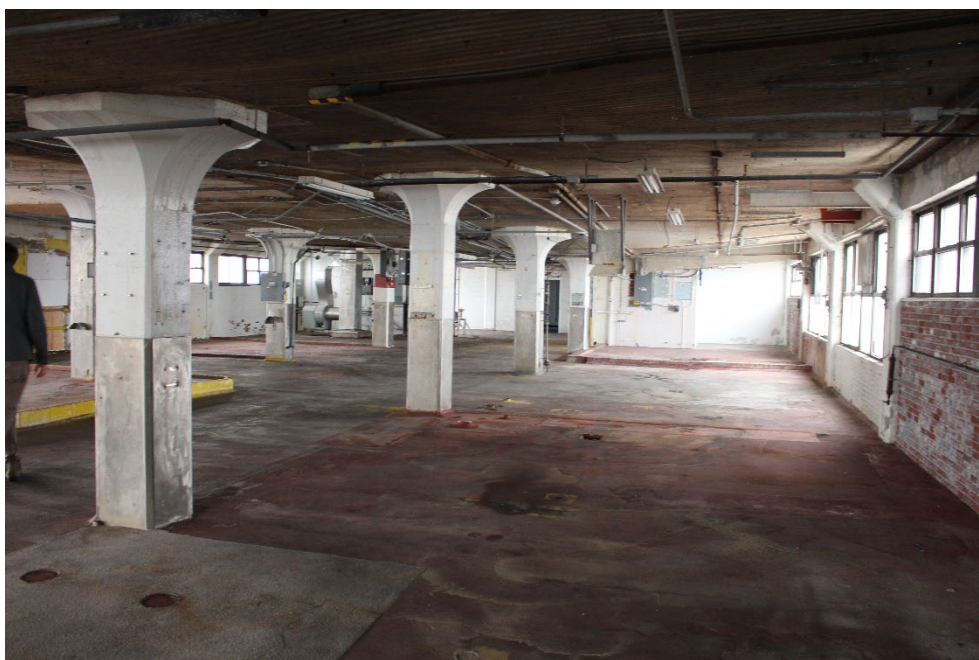
10. B&M Factory, Fourth Floor, looking south.
