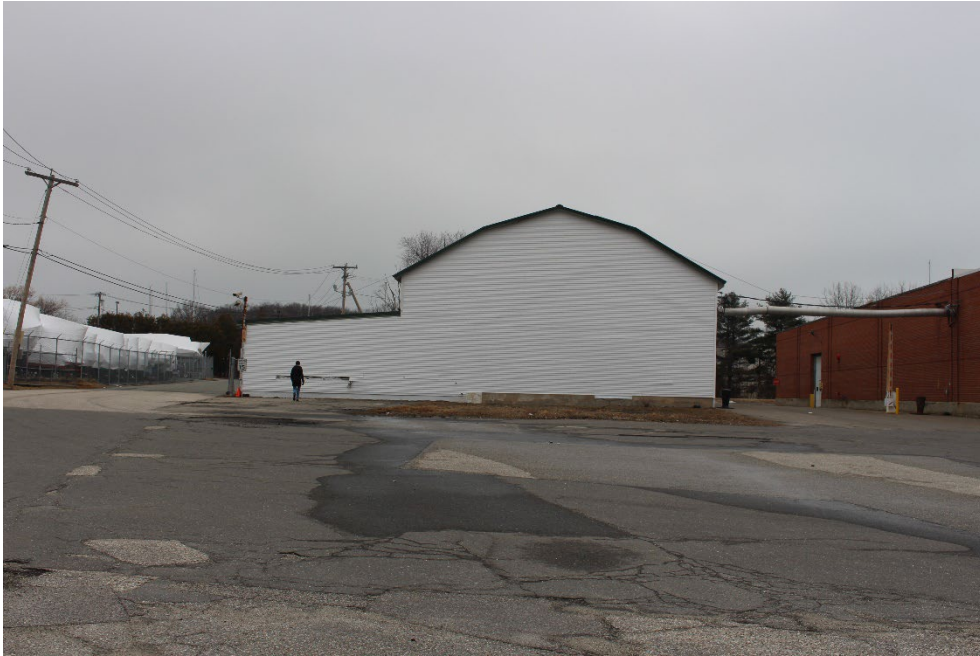
15. Site, Woodworking/Storage Building, looking northwest.
