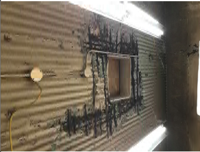
Photo 9 – Roof Slab Corrosion Deterioration
