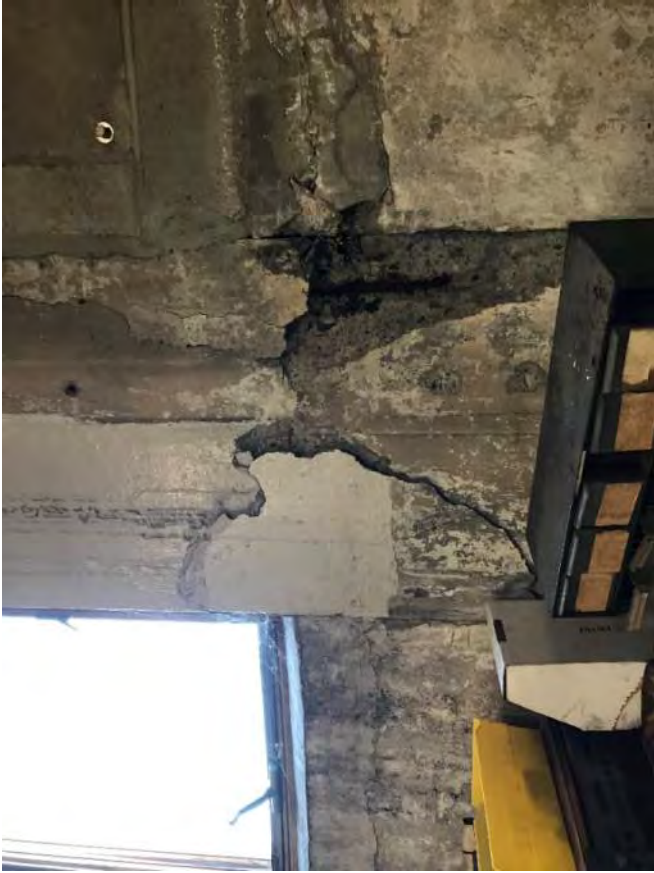
Photo 10 – Exterior Roof Column Corrosion Deterioration
