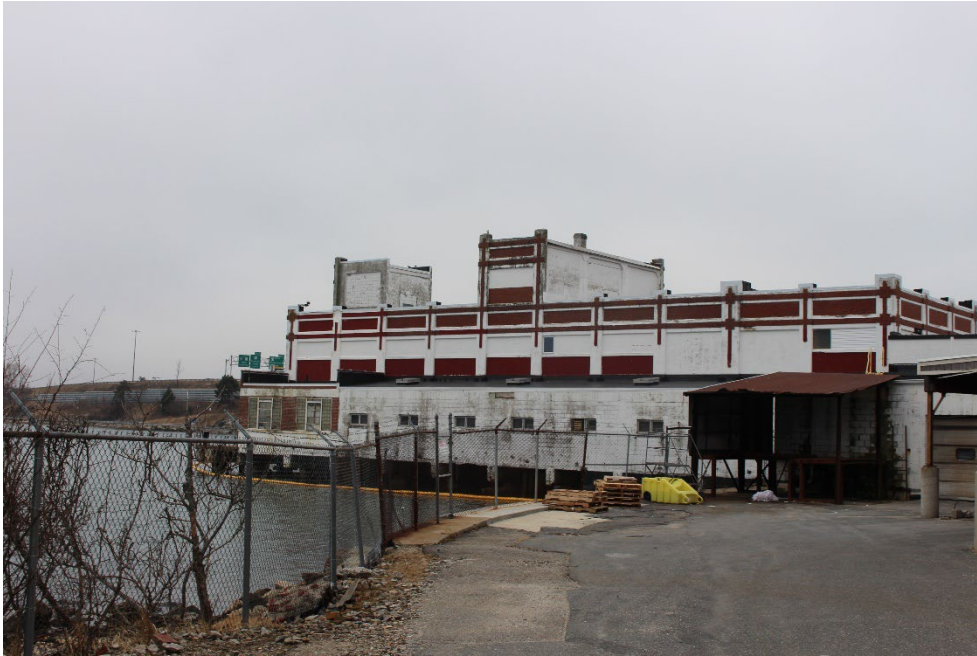
13. Site, Codfish Canning Building, looking southwest.
