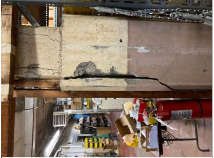
Photo 10 – Exterior Roof Column Corrosion Deterioration
