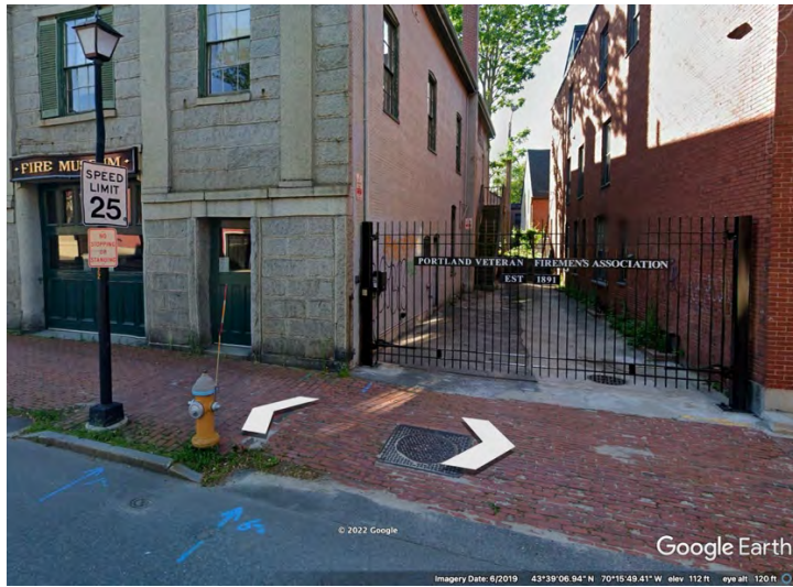
Figure 4 Gate at property's edge with no offset from sidewalk (recently completed)
