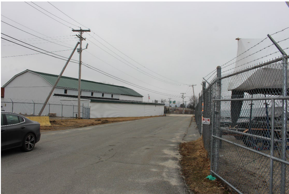
16. Site, Entrance and Woodworking/Storage Building looking south.
