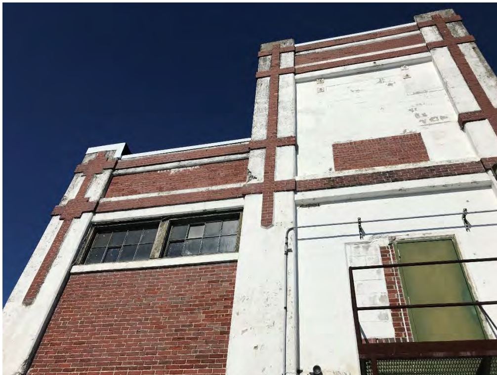
Photo 8. Maintenance Building. Exterior building condition.
