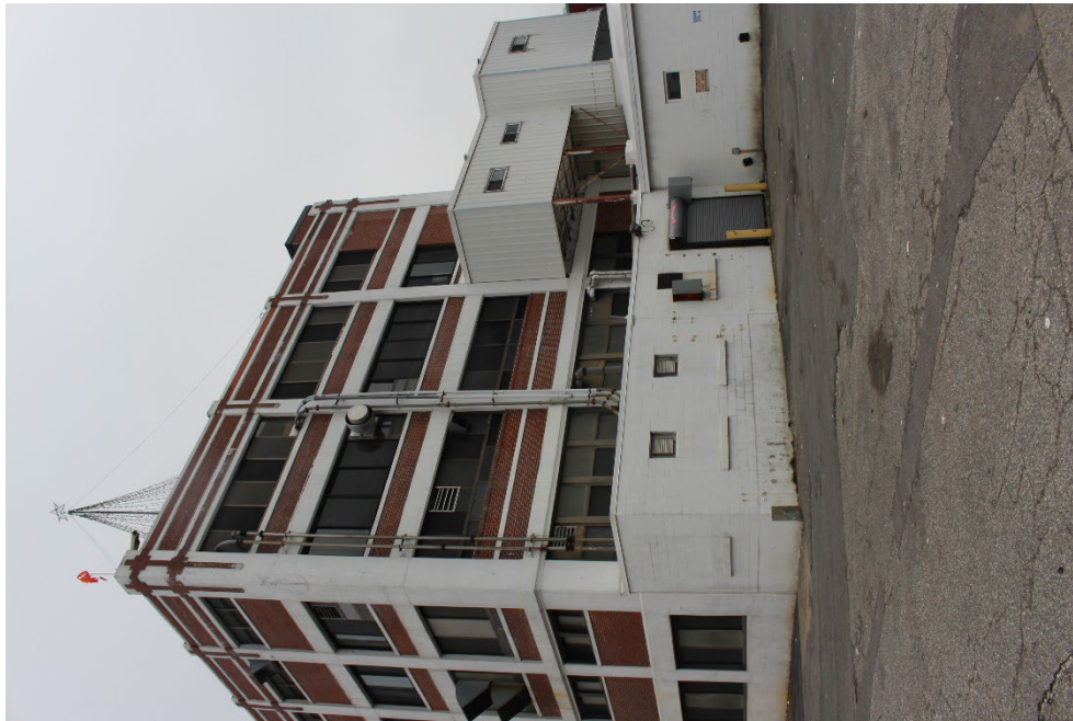
3. B&M Factory, South Elevation, looking north.
