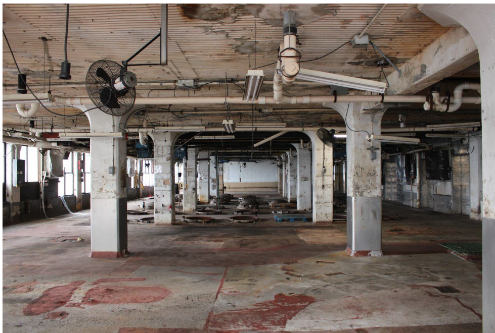
9. B&M Factory, Second Floor, looking north.
