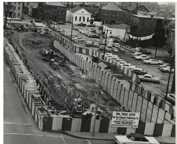
Figure 4: Western view of the subject property in 1965 showing the construction of the Portland Press Herald Printing Facility. The original alignment of Chapel Street can be seen in the portion of the site cordoned off for materials storage. Source: Maine Historical Society
