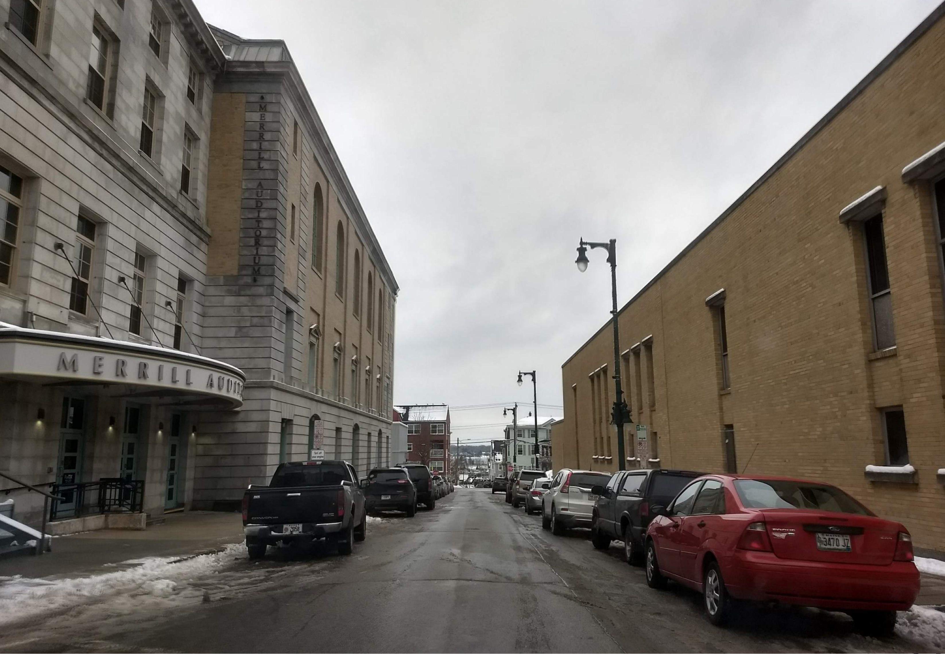
EXISTING CONDITIONS PHOTO
