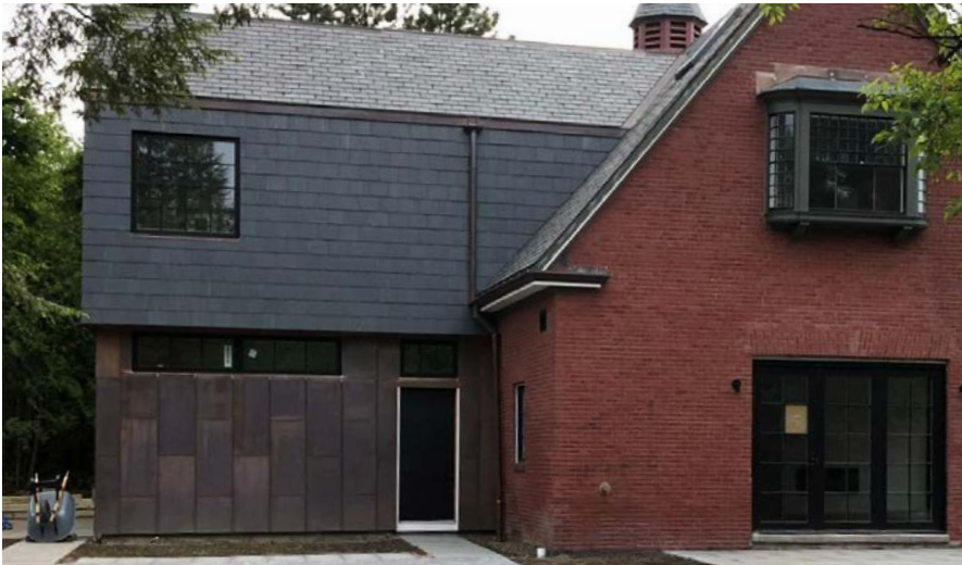
4. 188 Vaughan St - Walter D Davis Stable - Contemporary Addition Rhythm through paneling.
