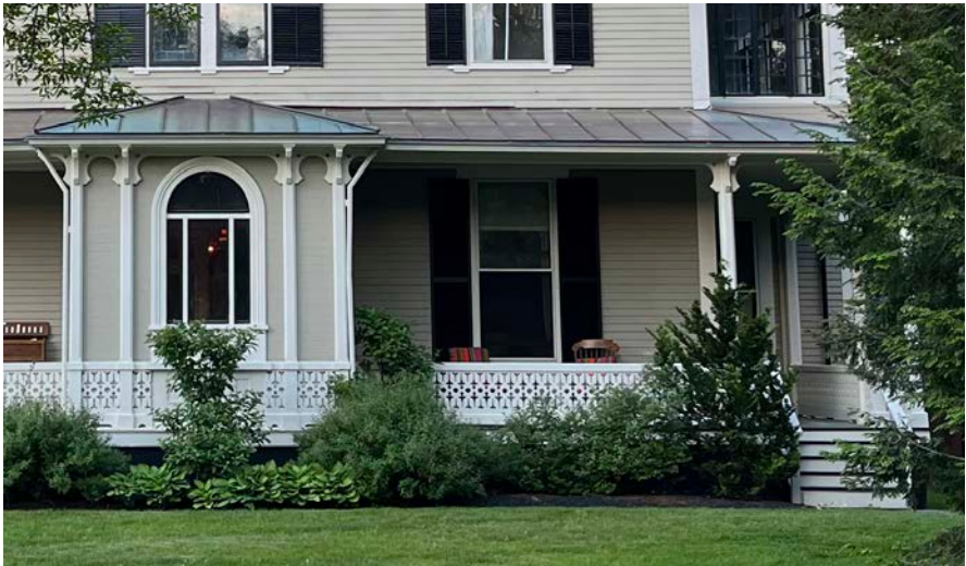
6. 113 Vaughan St - John Marshall Brown House - Italianate
