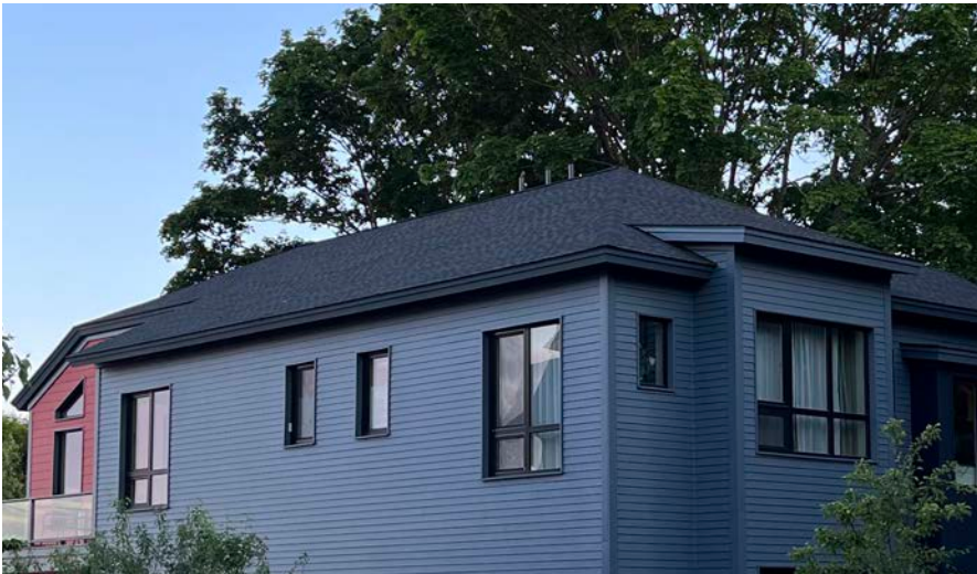
4. 382 Danforth St - Contemporary Single Family
