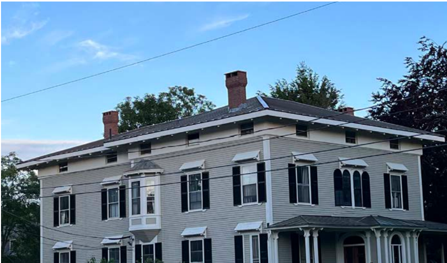
2. 113 Vaughan St - John Marshall Brown House - Italianate
