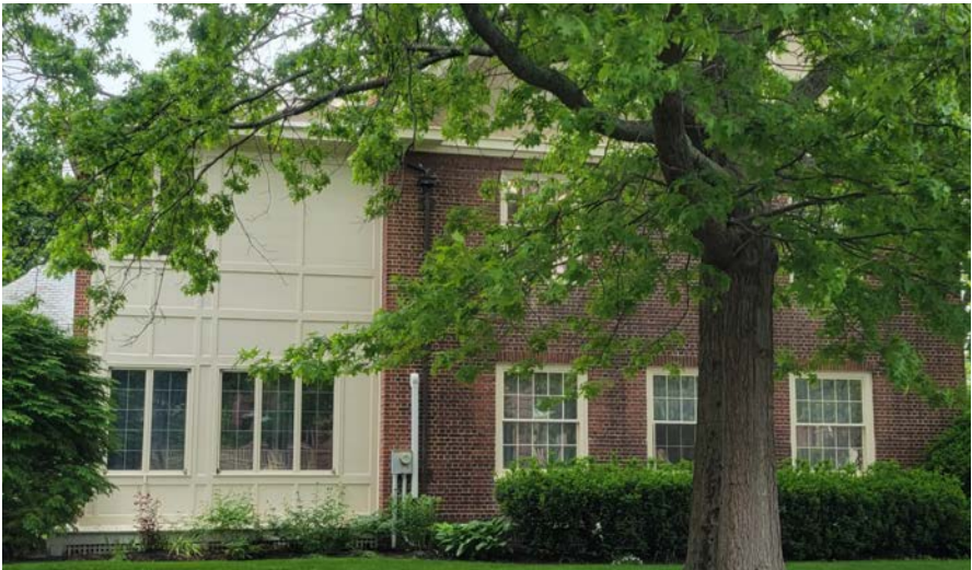
2. 71 Carroll St - Phillip G. Clifford House - Colonial Revival Vertical and Horizontal lines are generated from fenestration layout.
