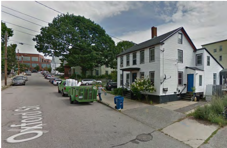
Figure 3 – Street View of Existing Building Facing Northeast
