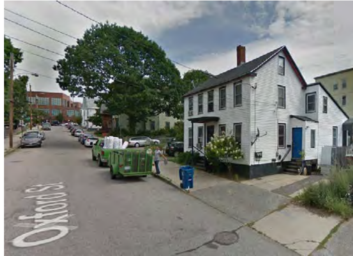
Figure 3 – Street View of Existing Building Facing Northeast
