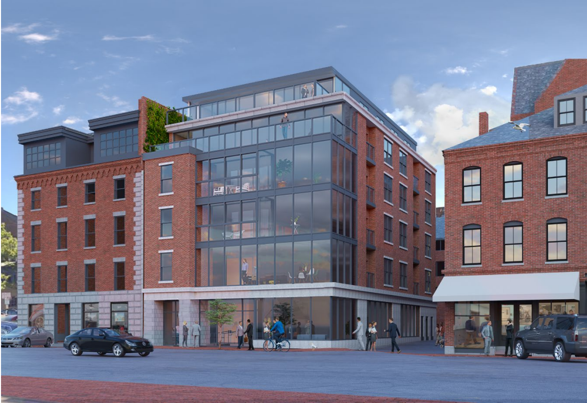
Current Design, Accordion Windows Closed:
