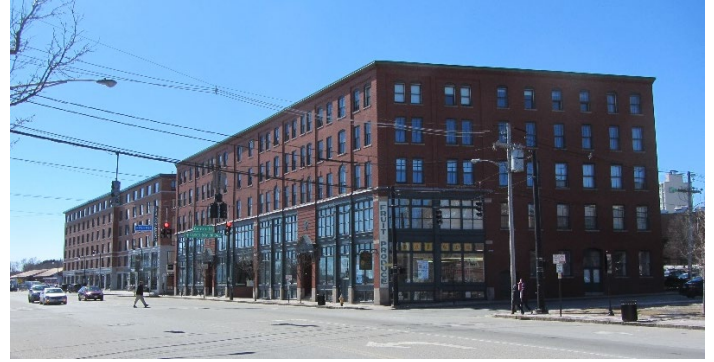
1902 Porteous warehouse in foreground and new construction beyond.
