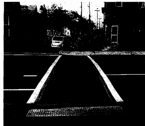
Highly visible, universally accessible crosswalk combining a detectable warning surface, brick pavers, granite bands, and paint. Crossing of Congress Street at North Street.
