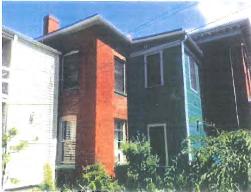
Image No.6 – rear of 147 Congress Street
