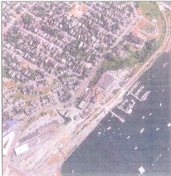
Figure 23, Aerial View of 58 Fore Street
