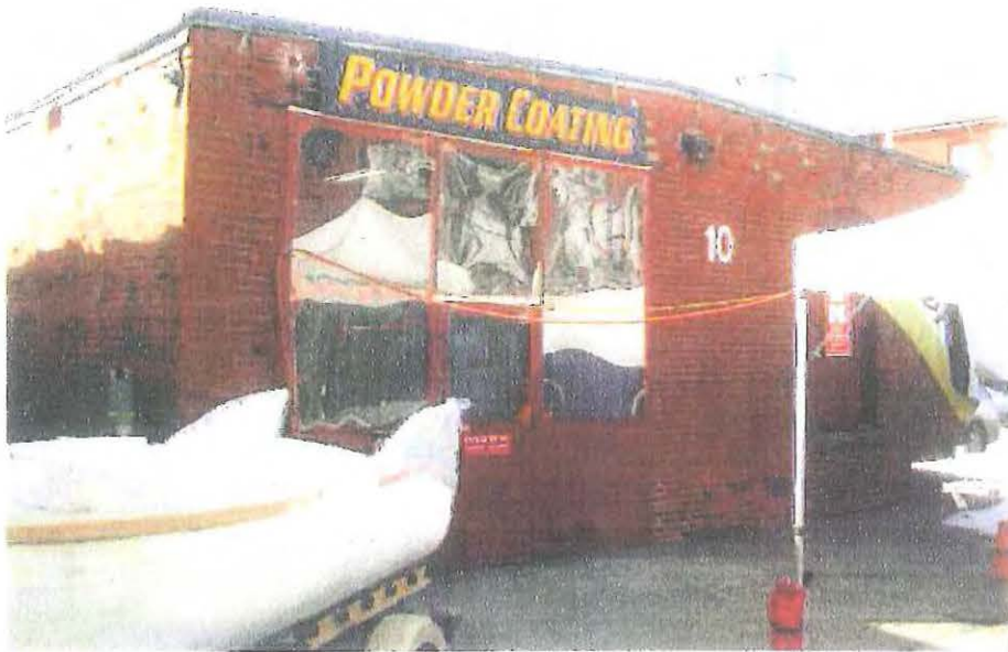
Photo 10-1: Exterior view of Building 10.
