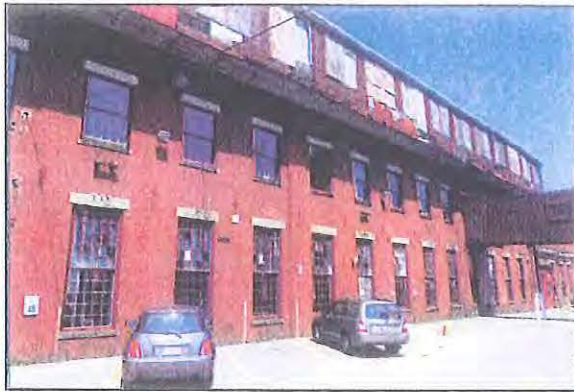
Building 2: Machine Shop Construction Date: c. 1847
