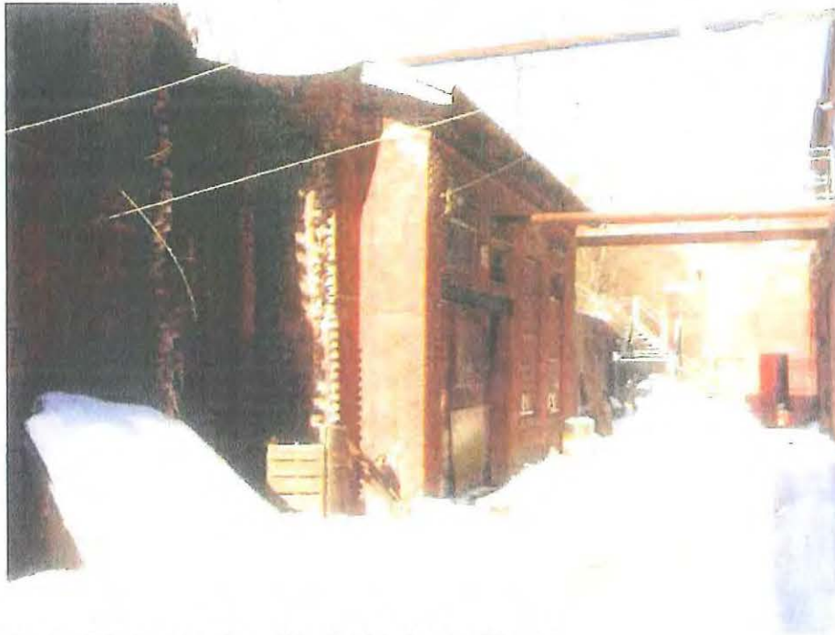
Photo 16-1: Exterior view of blacksmith shop/Building 16.
