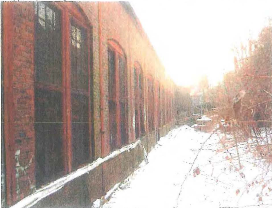
Photo 4-2: Exterior of Building 4, North Side.
