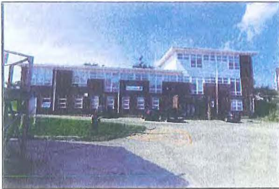
Building 30: Office Construction Date: 1950
