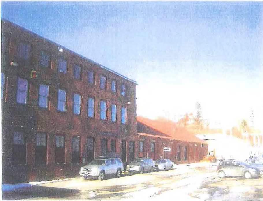
Photo 6B-1: Buildings 6A (left) and 6B (right).
