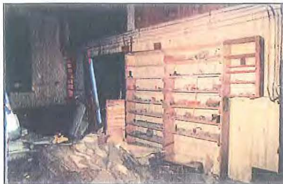
Current view of the lab/office space.
