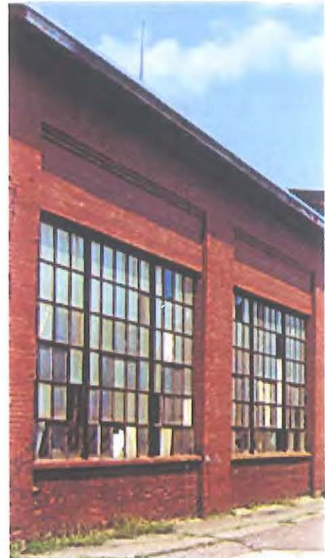
Windows within the manufacturing rows, whether on mid-19 th century structures or this 1918 Erecting Building, are typically large and multi-lite.
