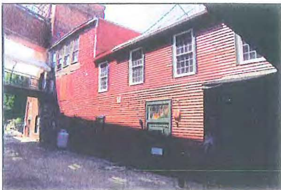
Building 14: Drafting Room and Storehouse Construction Date: 1858-64
