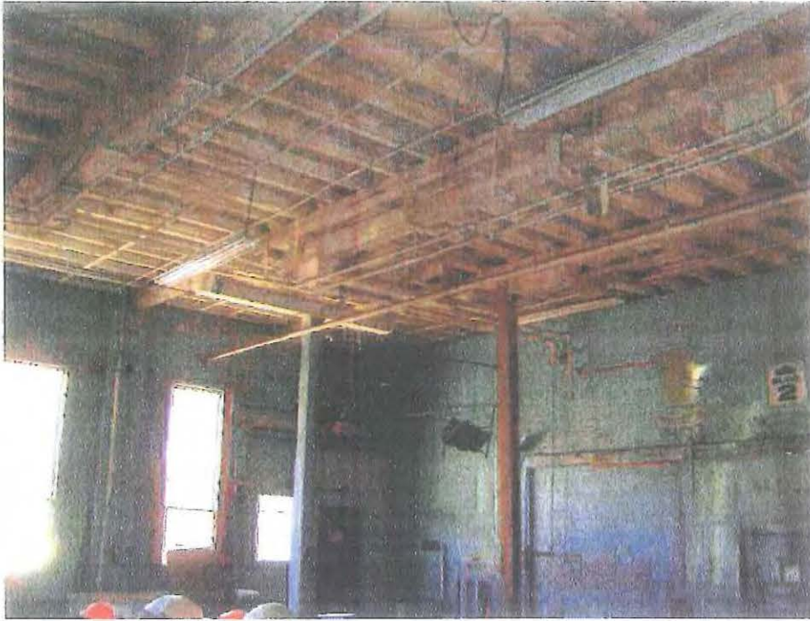
Photo 3-2: Interior view of Building 3. Note supplemental post, "T" column, queen post trusses.
