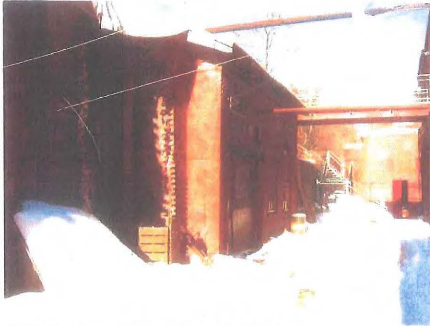
Photo 16-1: Exterior view of blacksmith shop/Building 16.
