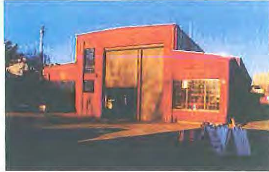
Building 1 – Erecting Shop, west Elevation
