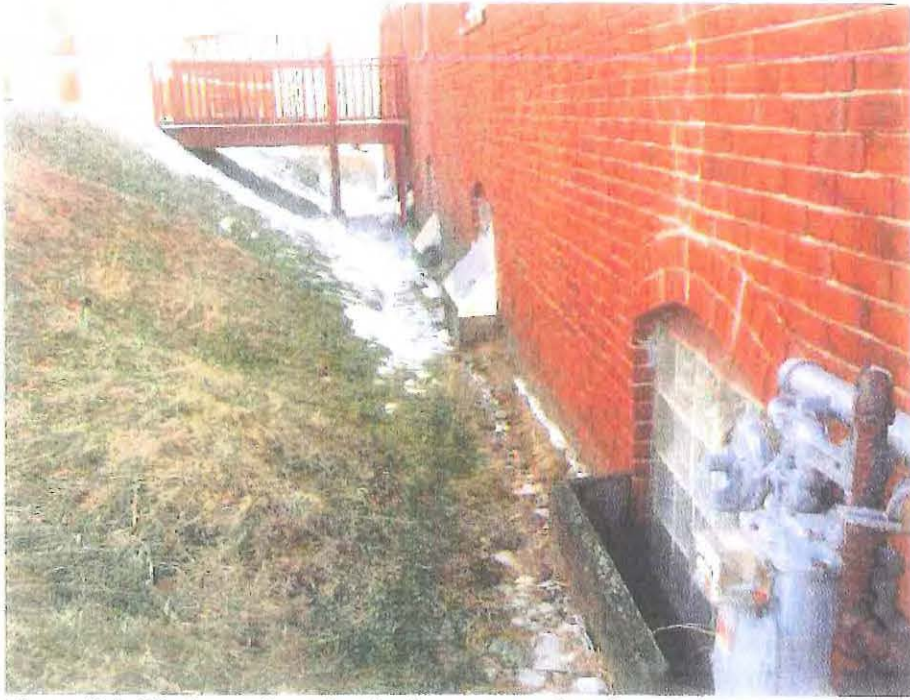
Photo 11-4: Window wells and embankment at north wall.
