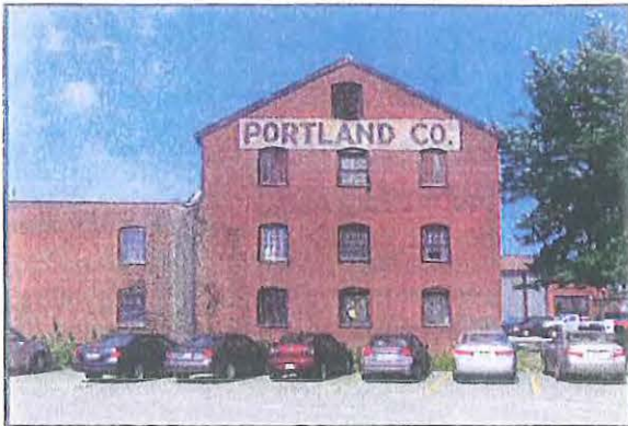
Building 12: Pattern Storehouse Addition Construction Date: 1895
