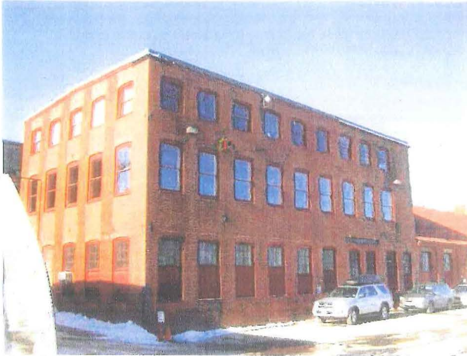
Photo 6A-1: Building 6A exterior view.
