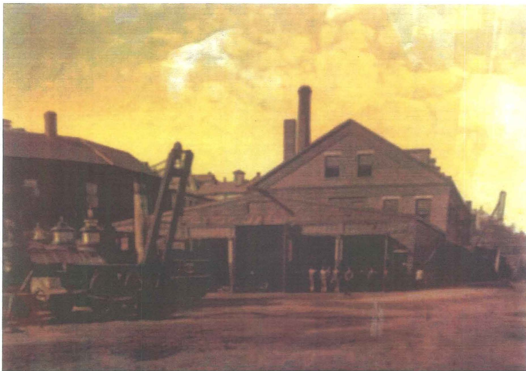
PHOTO B: Original version of Building 1 with low profile and no monitor built ~ 1880
