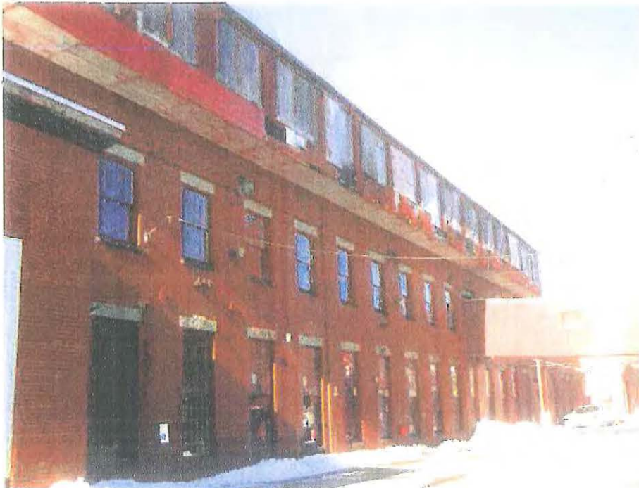
Photo 2-1: Building 2 exterior south elevation.
