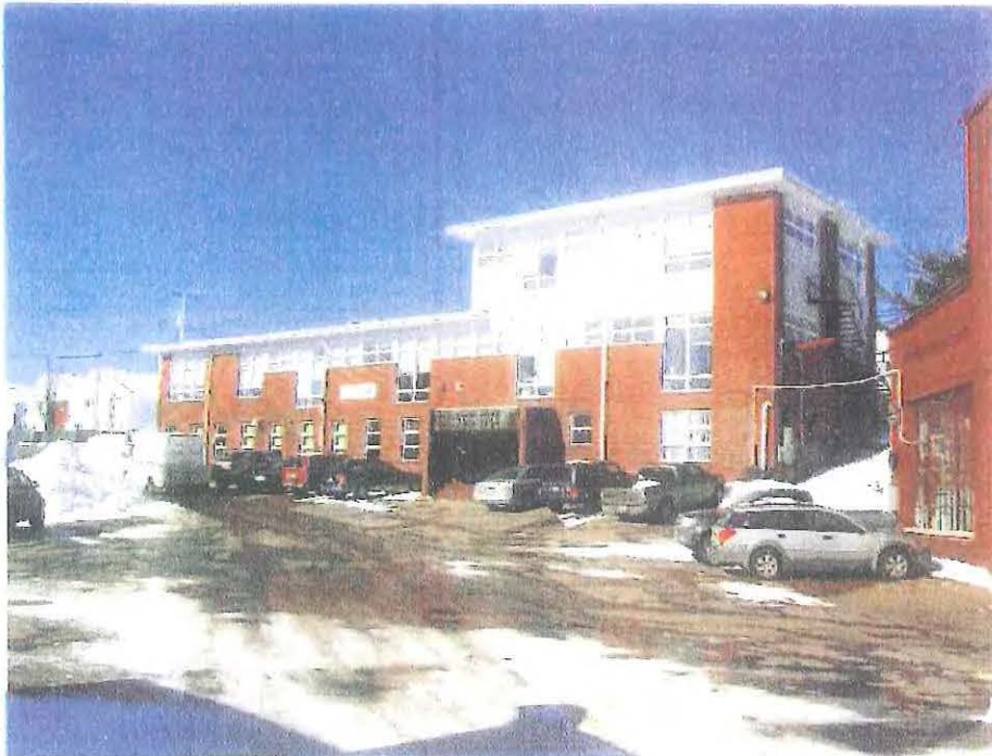
Photo 30-1: Southwest elevation of building 30.
