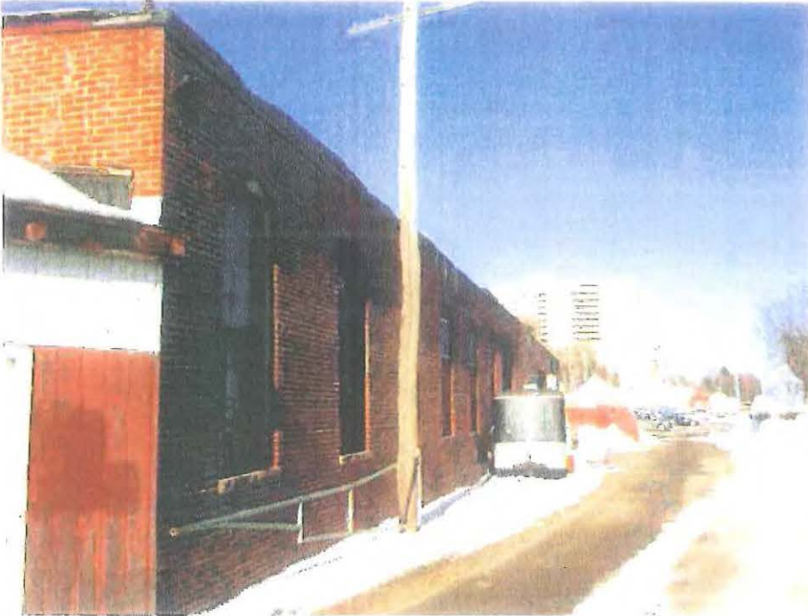
Photo 7-1: South elevation of Building 7.
