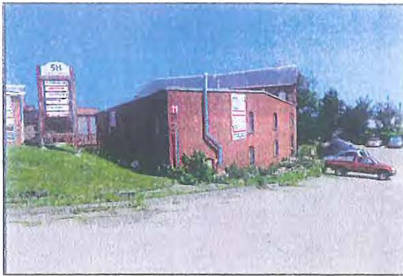
Building 11: Pattern Storehouse Construction Date: 1885; 1895
