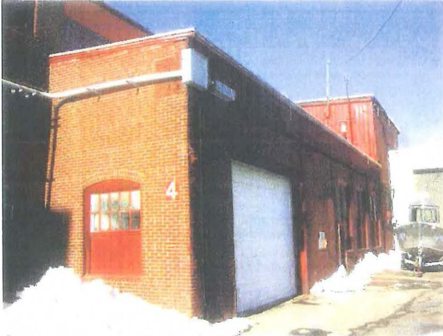
Photo 4-1: Exterior of Building 4. Note a majority of the south and east faces of the building are wrapped by Building 5.
