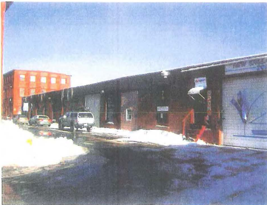
Photo 7-2: North elevation of Building 7.
