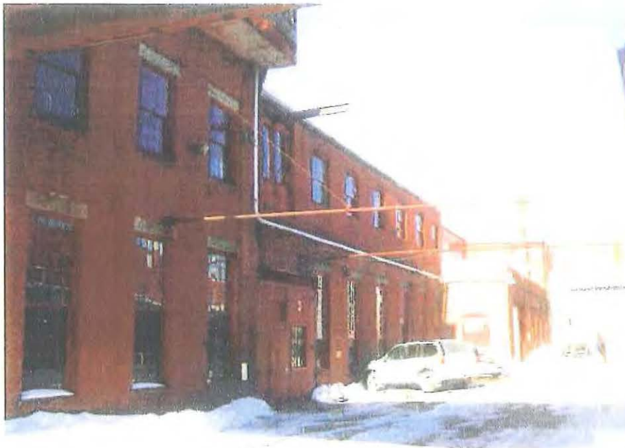
Photo 3-1: Exterior view of Building 3
