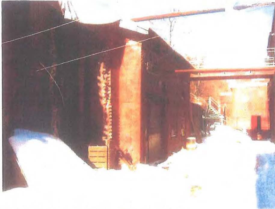
Photo 16-1: Exterior view of blacksmith shop/Building 16.
