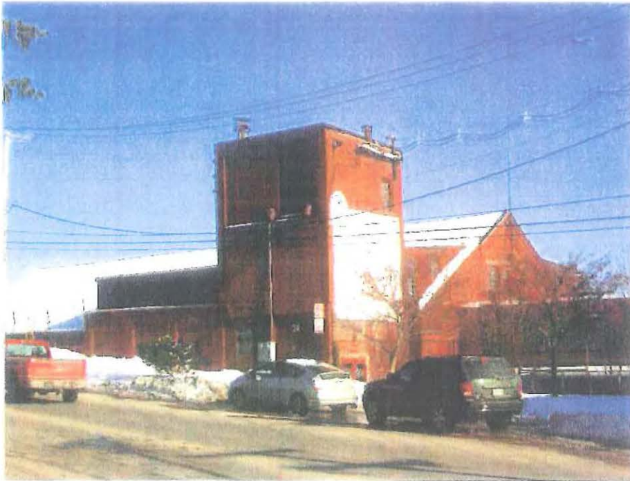
Photo 58-1: 58 Fore Street Vault/Tower structure viewed from Fore Street.
