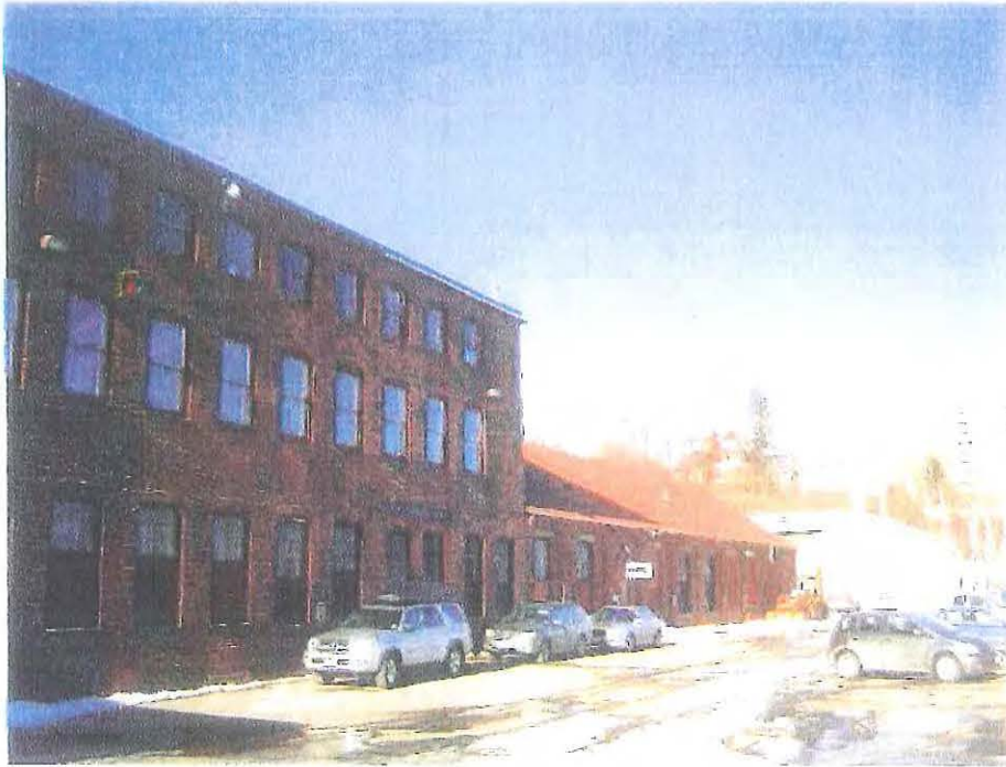
Photo 6B-1: Buildings 6A (left) and 6B (right).
