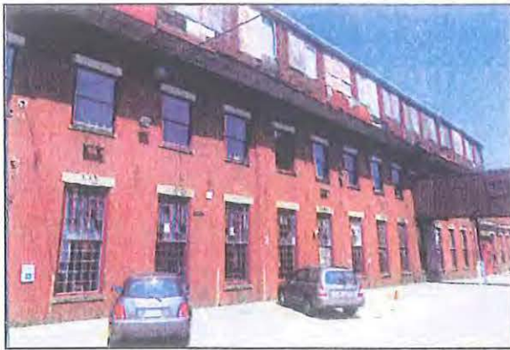
Building 2: Machine Shop Construction Date: c. 1847
