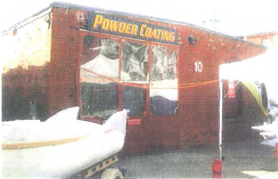
Photo 10-1: Exterior view of Building 10.
