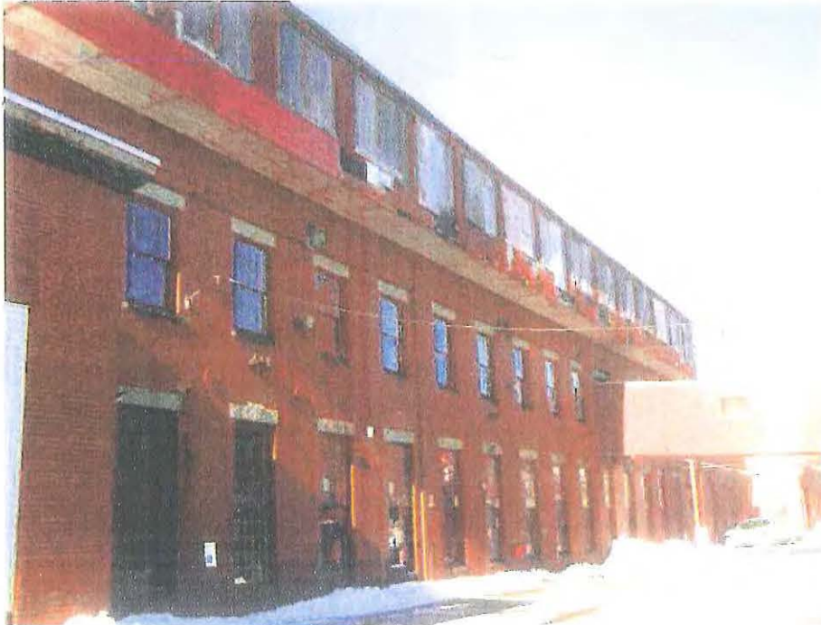
Photo 2-1: Building 2 exterior south elevation.
