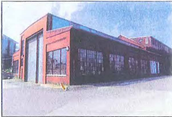
Building 1: Erecting Shop Construction Date: 1918
