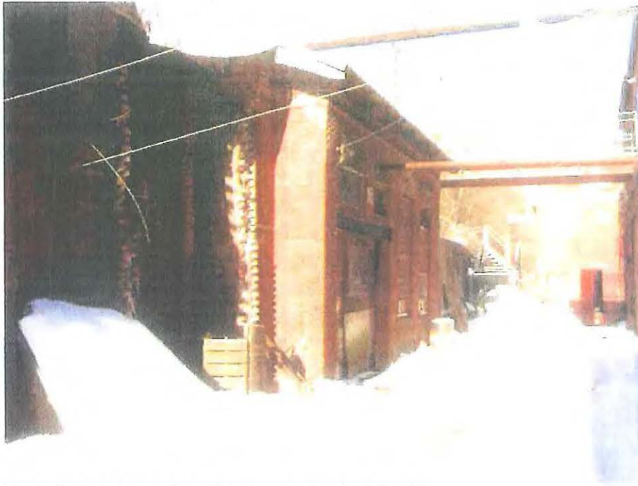
Photo 16-1: Exterior view of blacksmith shop/Building 16.
