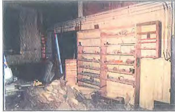
Current view of the lab/office space.
