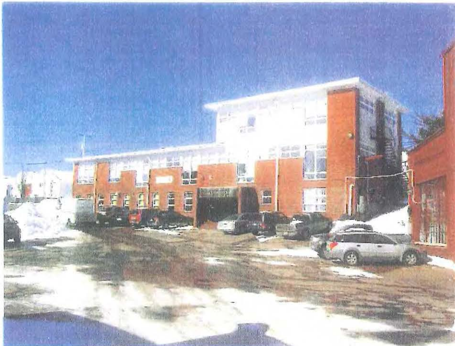
Photo 30-1: Southwest elevation of building 30.
