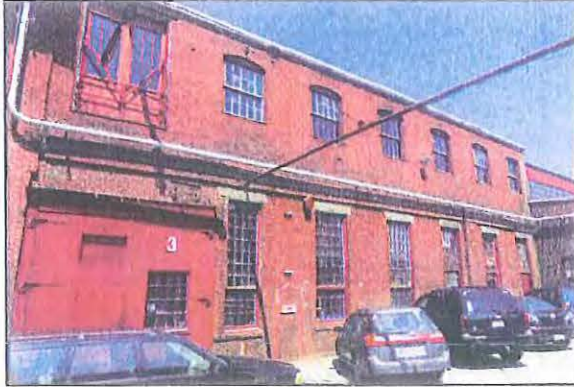
Building 3: Machine Shop Construction Date: c. 1847
