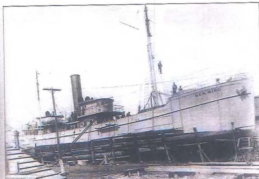
The nearly completed fishing trawler Sea Bird is still on the ways in the South Portland yard in 1919. She will be launched shortly after a few last-minute adjustments are finished. The 163-foot trawler weighed 383 gross tons and was built for the East Coast Fisheries Company of Portland, Maine.
