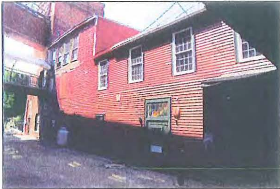
Building 14: Drafting Room and Storehouse Construction Date: 1858-64
