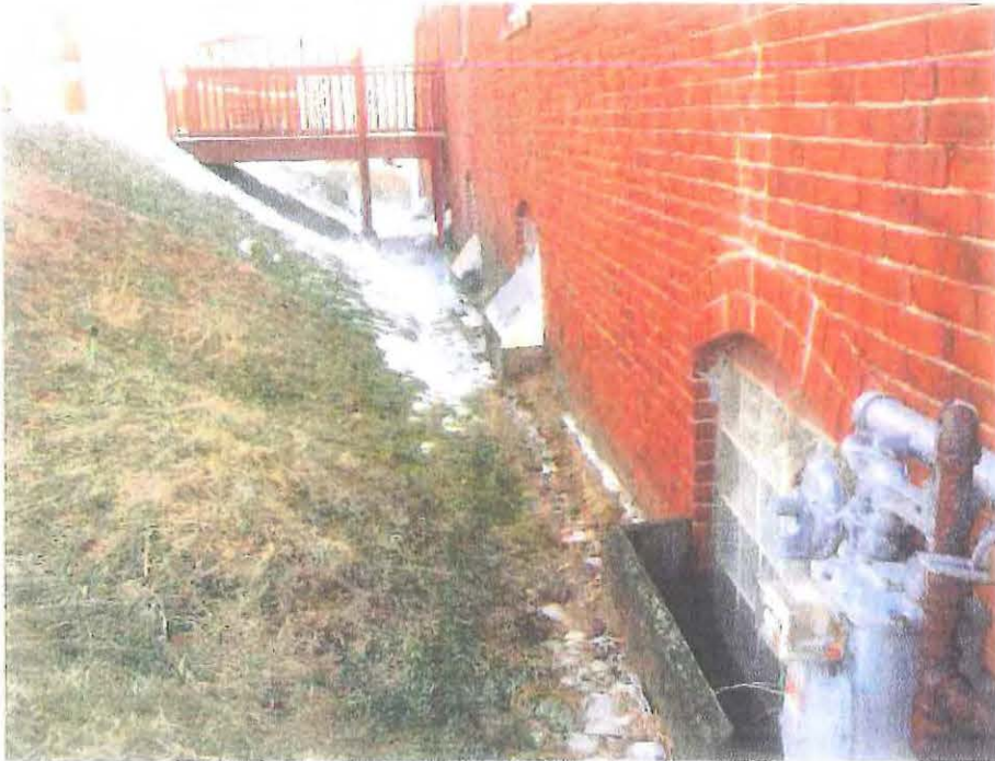
Photo 11-4: Window wells and embankment at north wall.
