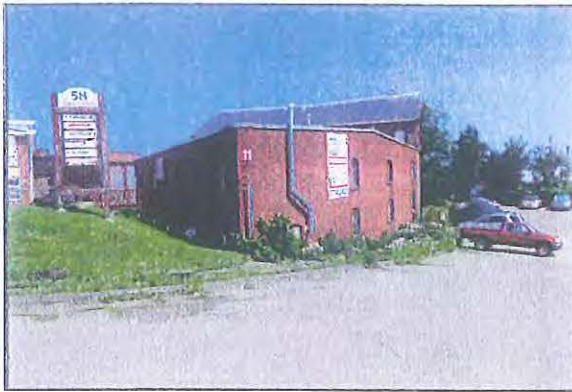
Building 11: Pattern Storehouse Construction Date: 1885; 1895
