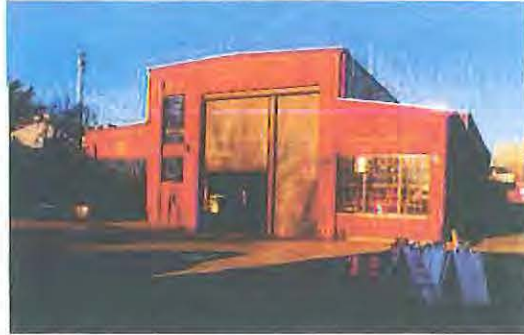
Building 1 – Erecting Shop, west Elevation
