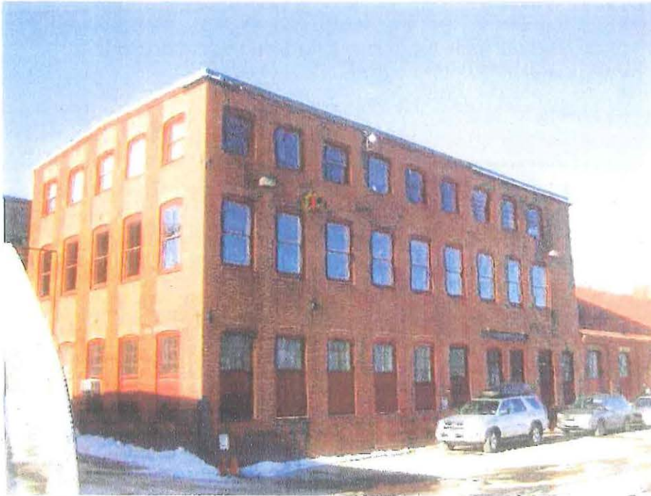
Photo 6A-1: Building 6A exterior view.
