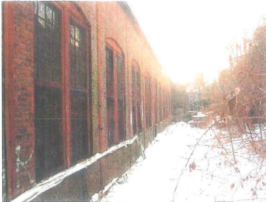
Photo 4-2: Exterior of Building 4, North Side.
