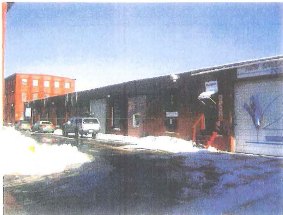
Photo 7-2: North elevation of Building 7.
