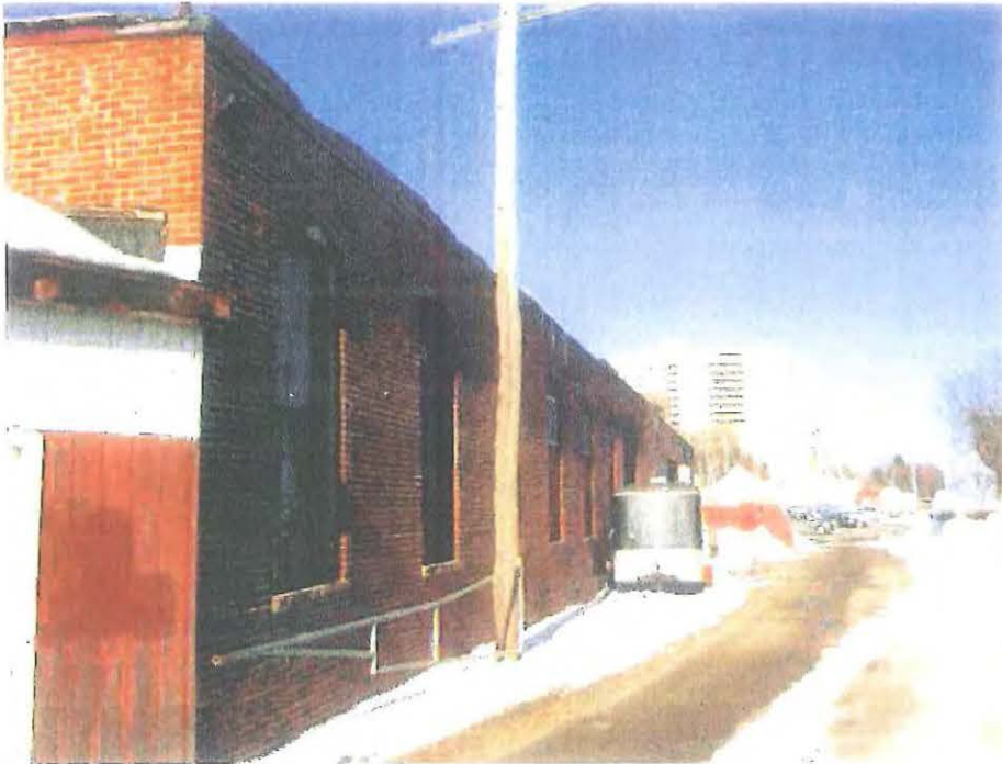
Photo 7-1: South elevation of Building 7.
