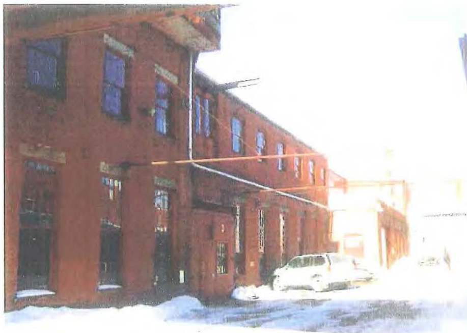
Photo 3-1: Exterior view of Building 3
