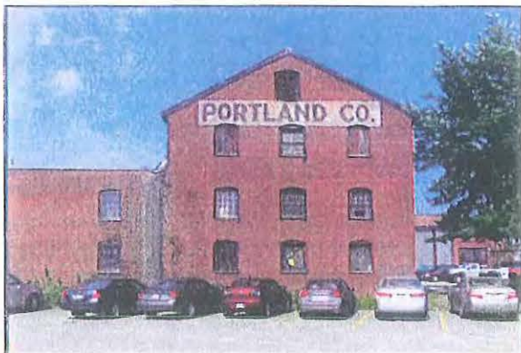
Building 12: Pattern Storehouse Addition Construction Date: 1895
