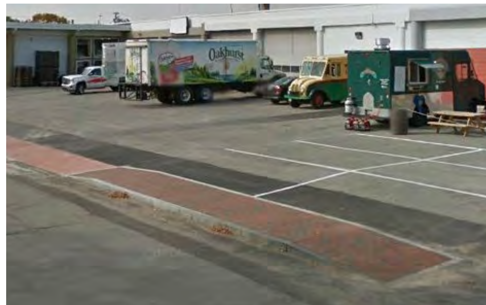
Figure 5-39: Fox Street after driveway improvements
