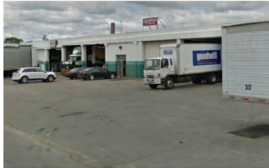
Figure 5-38: Fox Street before driveway improvements
