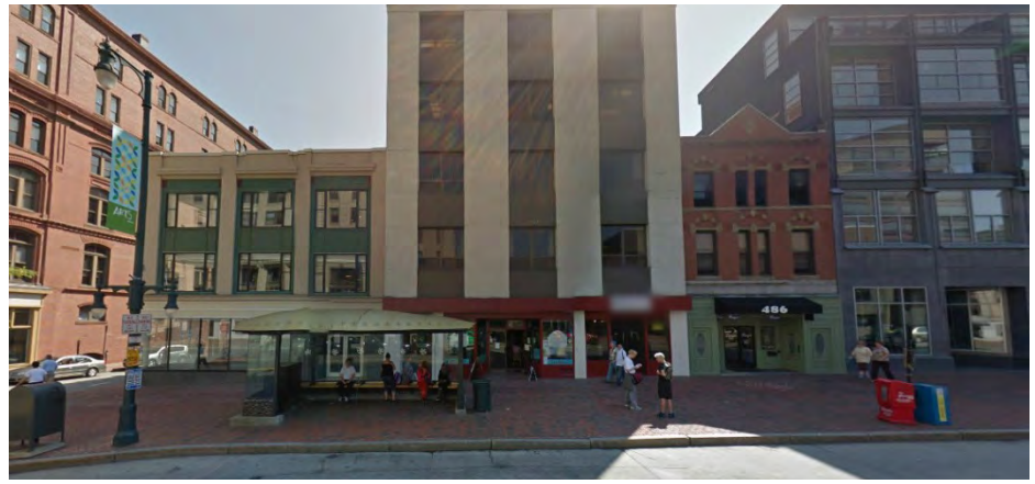
Figure 2-29: An existing bus stop that serves as a good example for Bayside is the Monument Square stop on Congress Street. This bus stop, located within a bus pull out, or bus bay, has sufficient length for buses to pull out of the travel lane and to the curb. Rider amenities include a shelter, bench, and trash receptacle. The sidewalk adjacent to the stop is 25 feet wide and provides a level landing area (five feet wide by eight feet deep area at the front door zone). Crosswalks with curb ramps are provided in close proximity to the stop.
