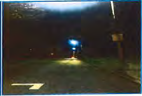
Baltimore After – LED Cobra Head Luminaires
