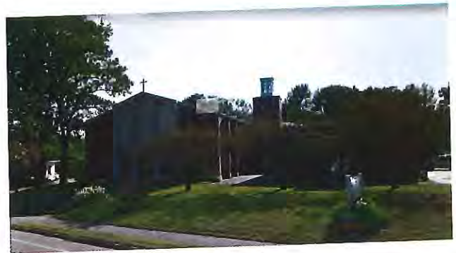
Figure 7: First Lutheran Church
