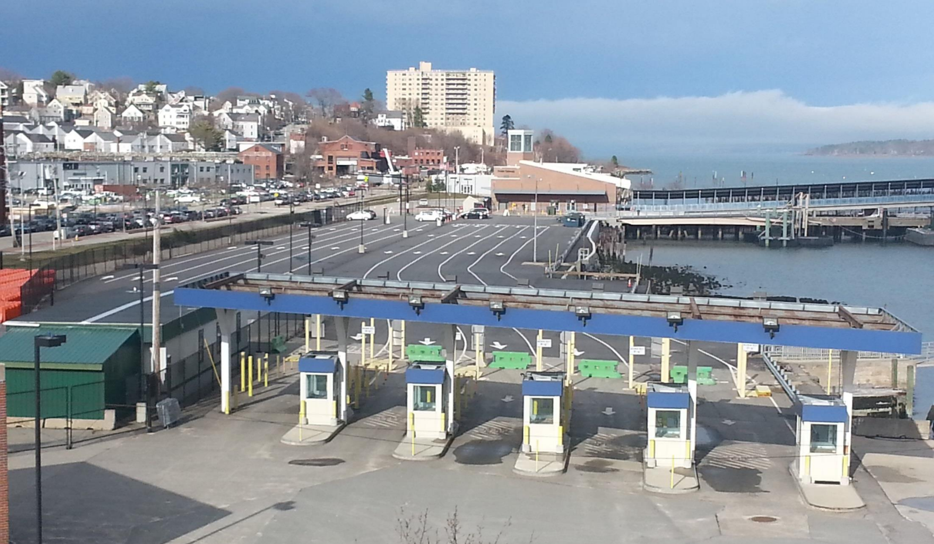
Ocean Gateway queuing: current condition
