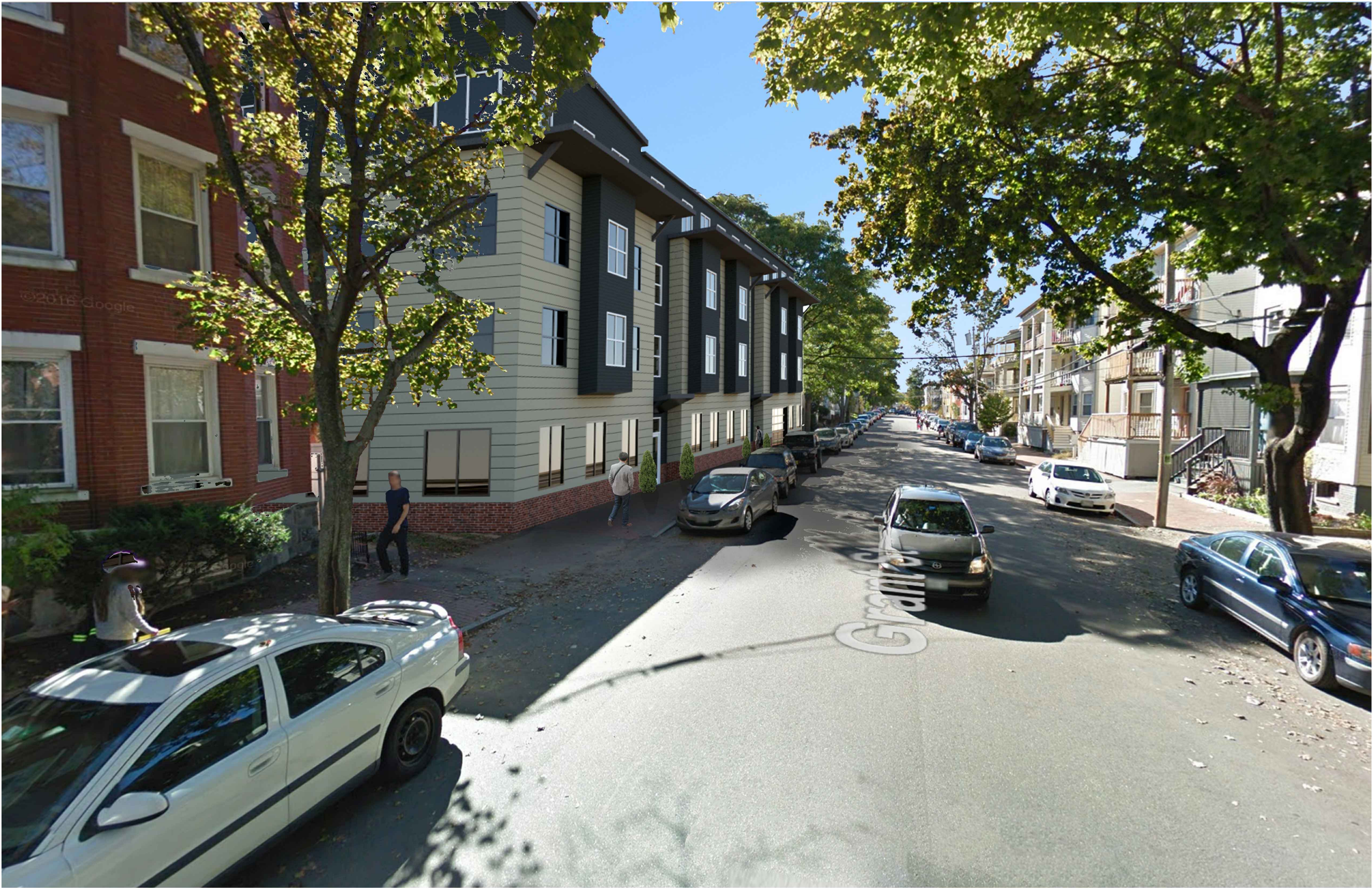
1 VIEW LOOKING WEST ON GRANT STREET N.T.S.
