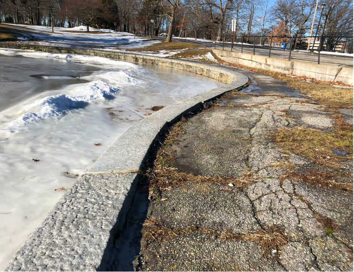
View of existing pond edge and retaining wall with railing.
