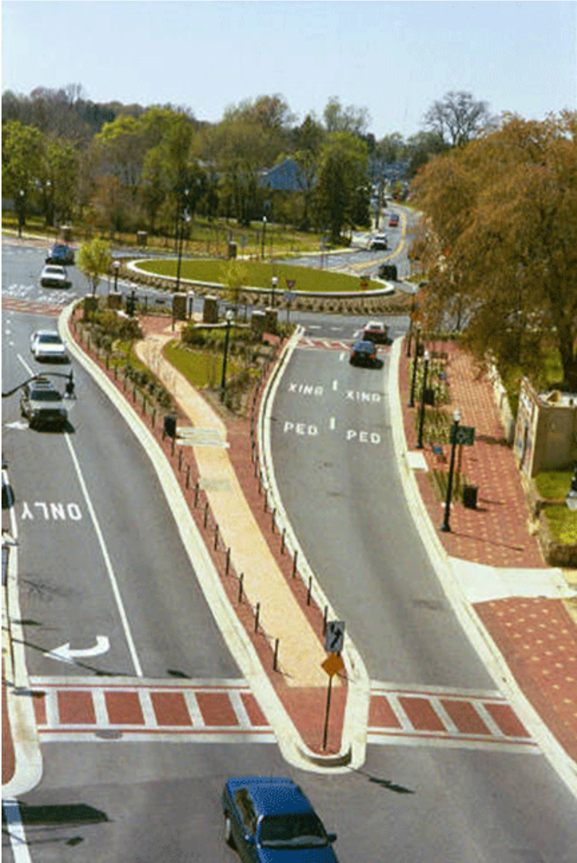
Annapolis, MD - 2 lane roundabout Century Engineering http://www.centuryeng.com/transgatewaycr.html
