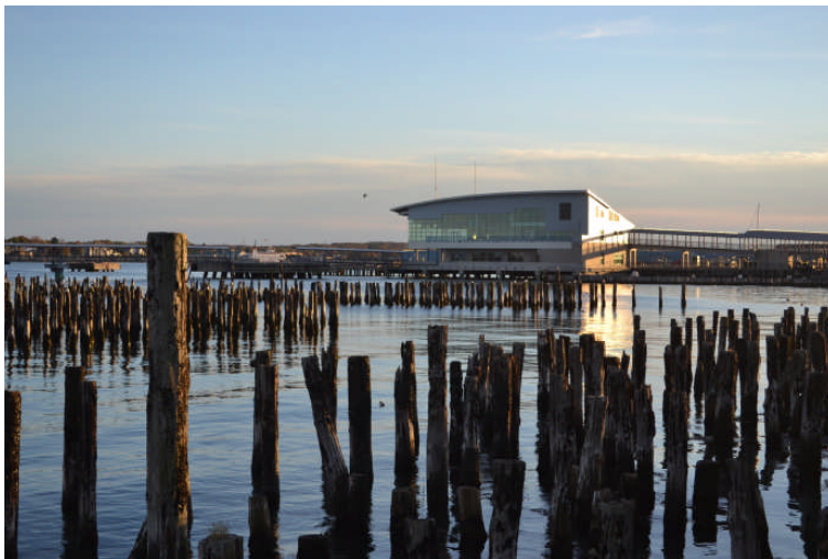
Figure 7.13 EXISTING GRAND TRUNK RR FIRE PIERS
