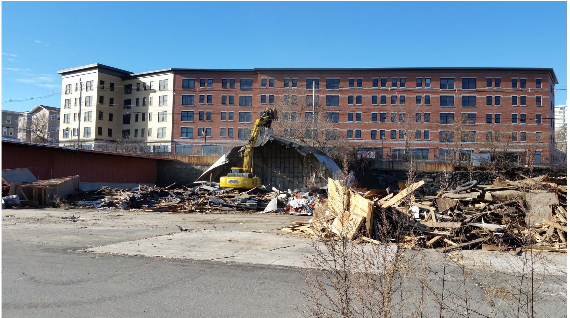
#15 Rufus Deering Site Demolition December 2018
