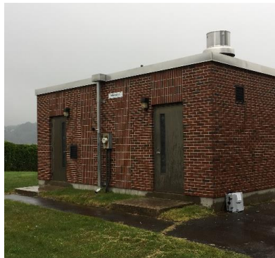
Location 14: Mechanic Street Pump House (South Portland)
