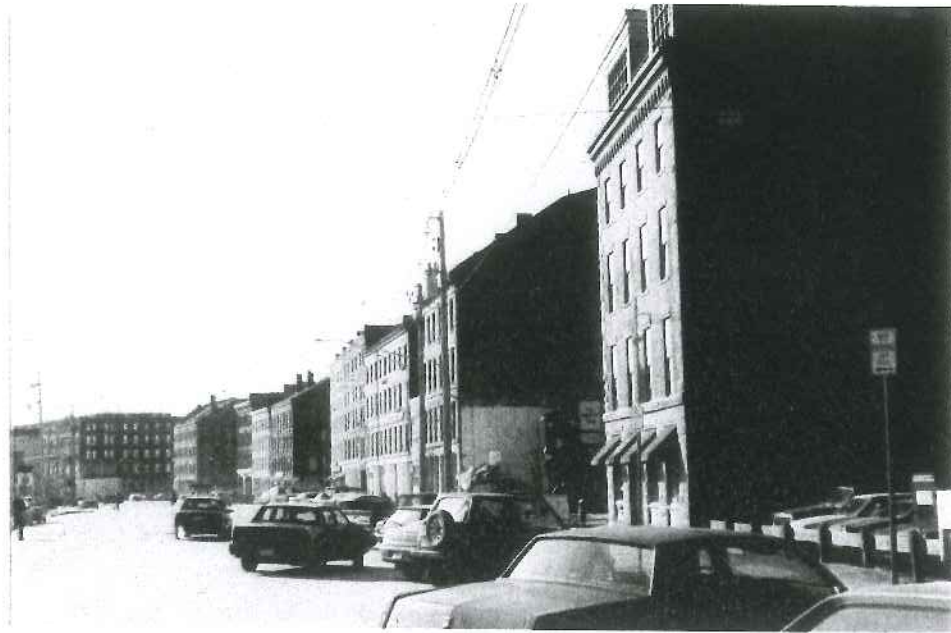
One of Portland's finest commercial "walls" is along Commercial Street. Here, commercial buildings of remarkably consistent character form the sides of the street for a number of blocks. Buildings of various sizes are grouped together in the traditional fashion to create the solid street facade out of many parts. The result is a sense of place and enclosure that is a uniquely urban and plays a major role in the "feel" of the Old Port.
