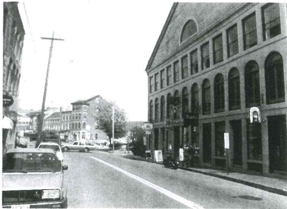
South side of Fore Street.
