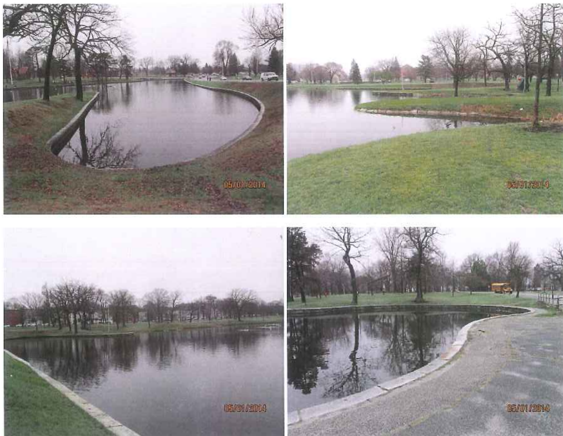
Figure 2-1 Deering Oaks Pond Existing Conditions Photographs
