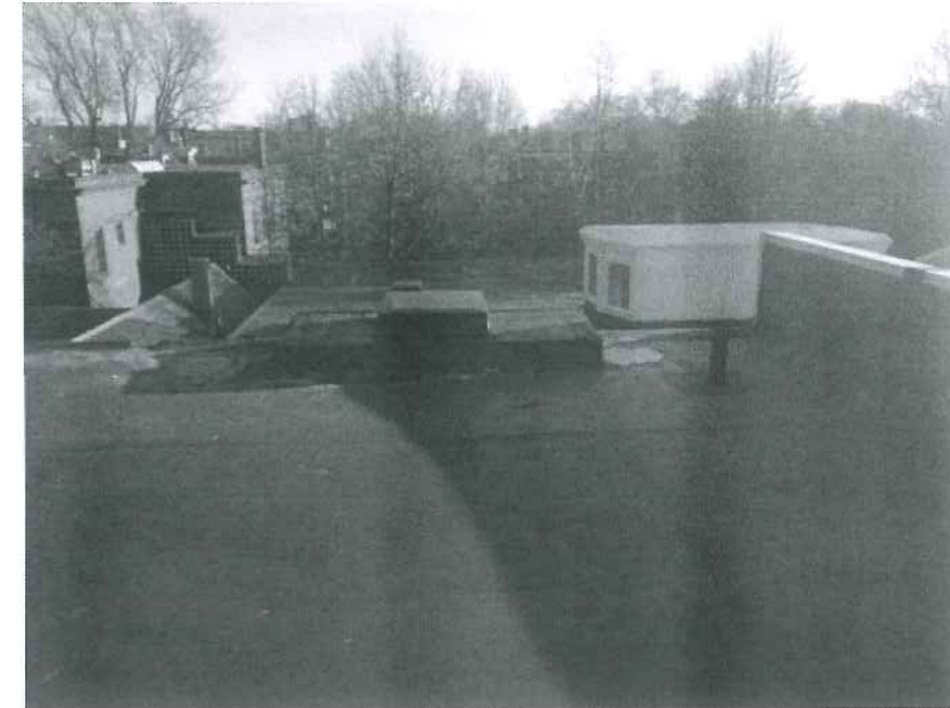
EXISTING CONDITION | LOOKING TOWARDS EXISTING HATCH
