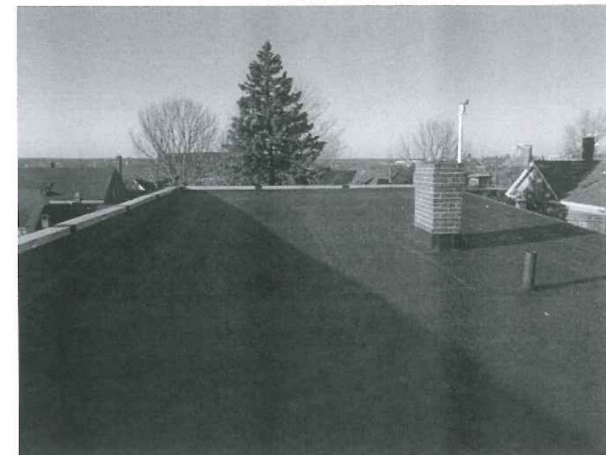
EXISTING CONDITION | FACING BRACKETT STREET
