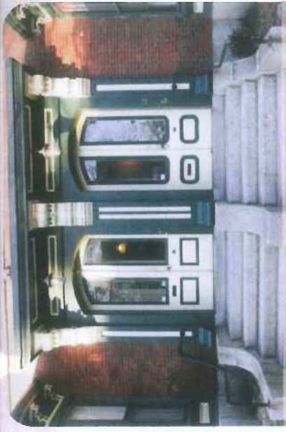
Image 21: Granite staircase & entrance 57-59 Deering Street
