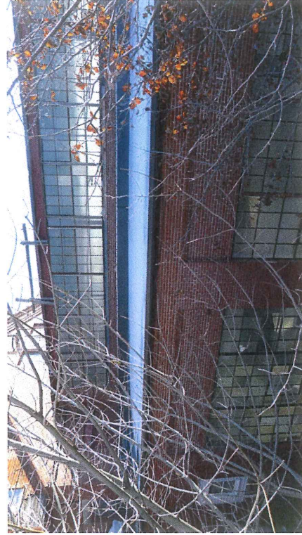
8 west elevation - detail of roof monitor
