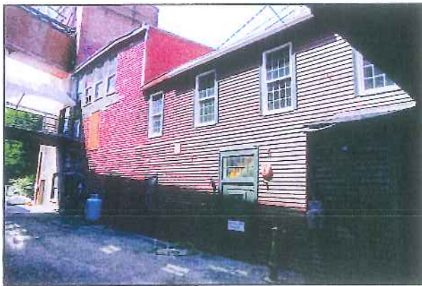
Building 14: Drafting Room and Storehouse Construction Date:
