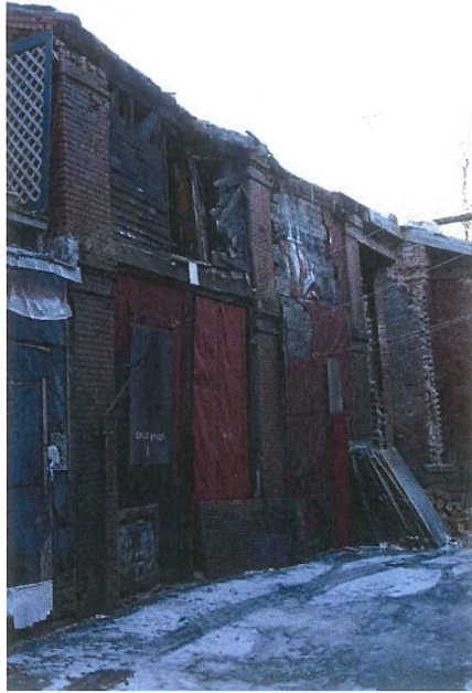
2 | east elevation - south end of Building 15
