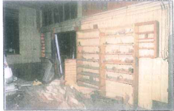
Current view of the lab/office space.
