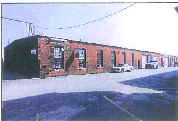
Building 7: Car Shop Construction Date:
