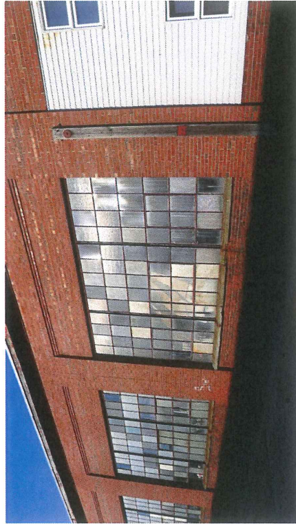
4 east elevation - detail at north end
