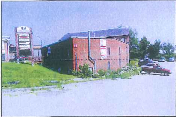
Building 11: Pattern Storehouse Construction Date: 1885; 1895
