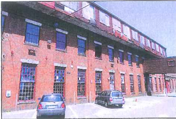
Building 2: Machine Shop Construction Date: c. 1847
