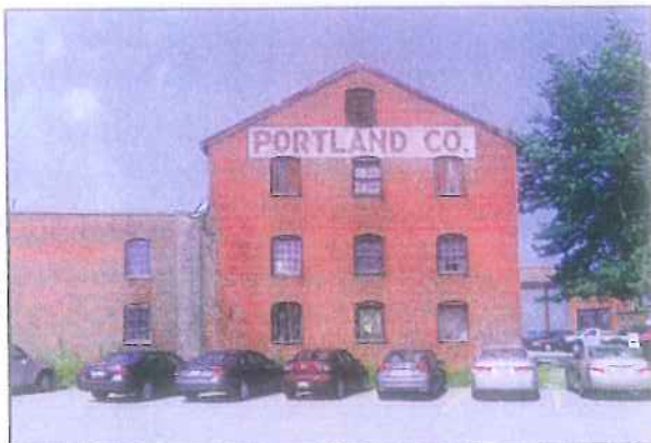
Building 12: Pattern Storehouse Addition Construction Date: 1895
