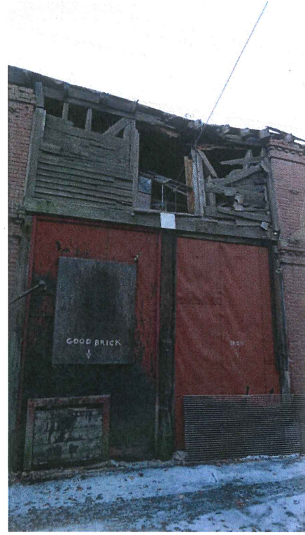
3 | east elevation - north end of Building 15
