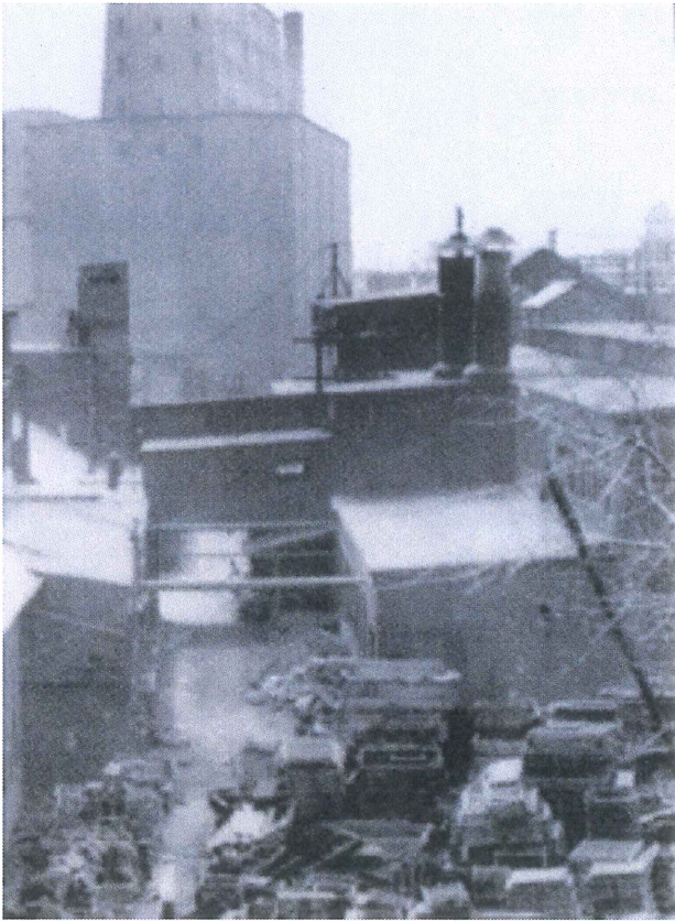
Building 4 (right) prior to demolition of Boiler House (left), which was later replaced by the existing Building 5
