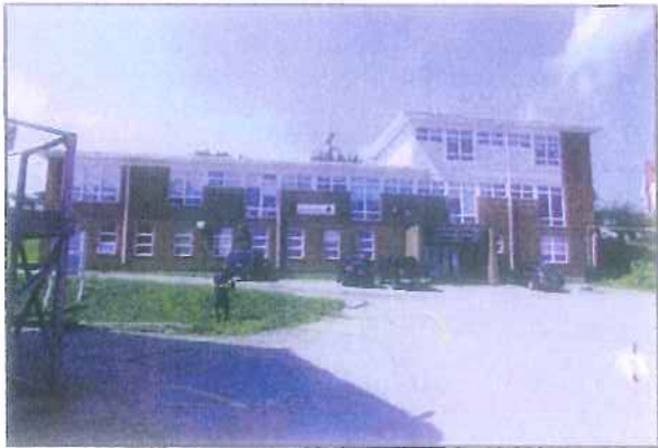
Building 30: Office Construction Date: 1950
