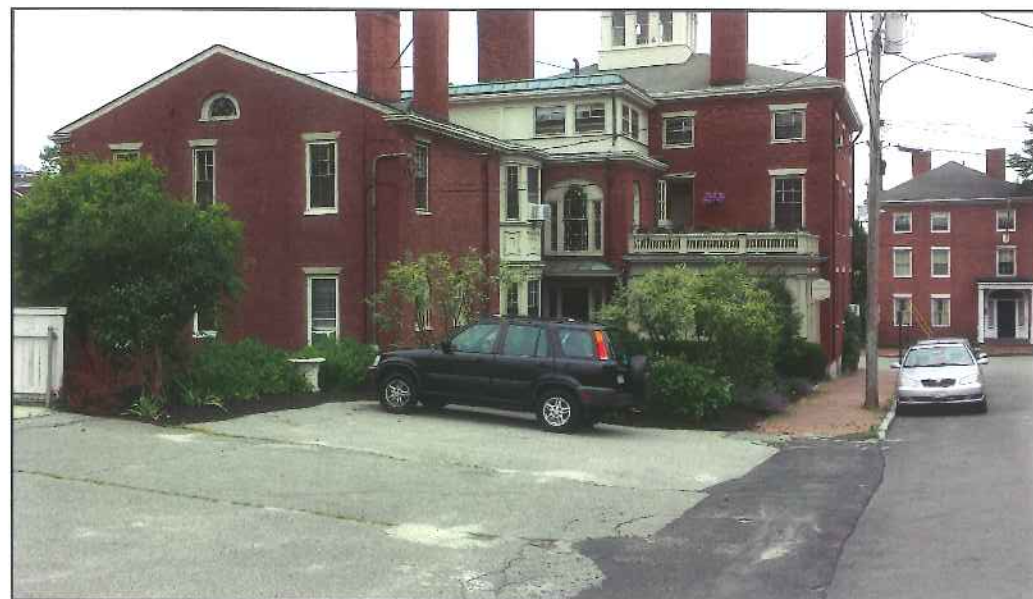
2 SK-3 EXISTING EXTERIOR CONDITIONS VIEW FROM SOUTHWEST (WINTER ST) SCALE: N/A
