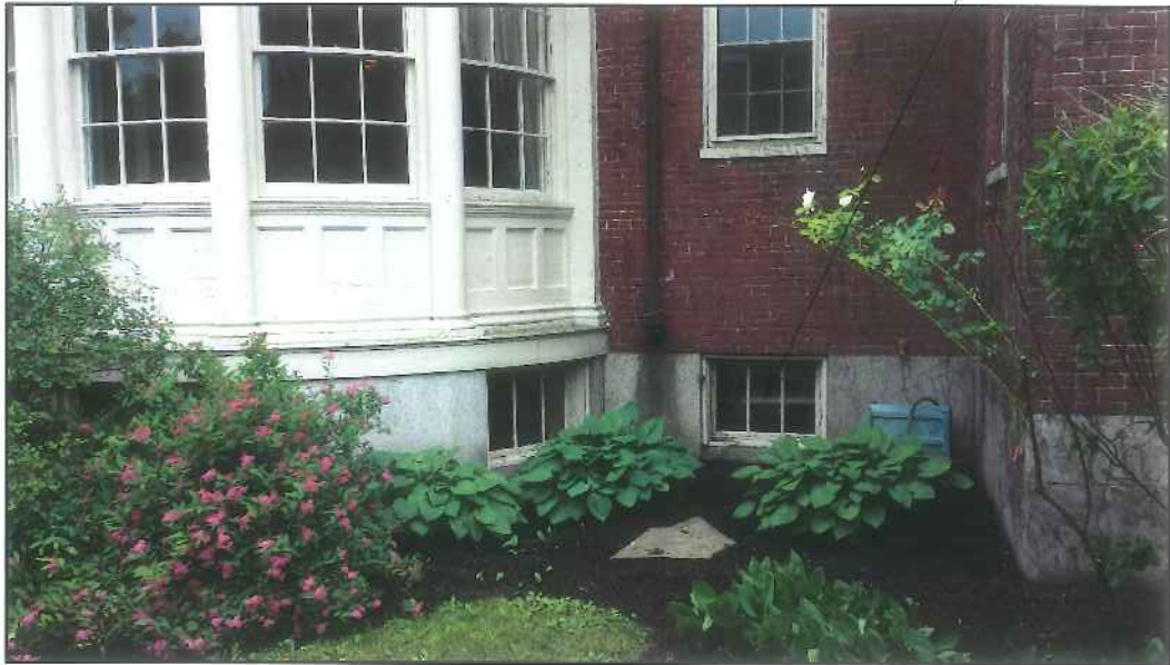
1 EXISTING EXTERIOR CONDITIONS SK-2 SCALE: N/A
