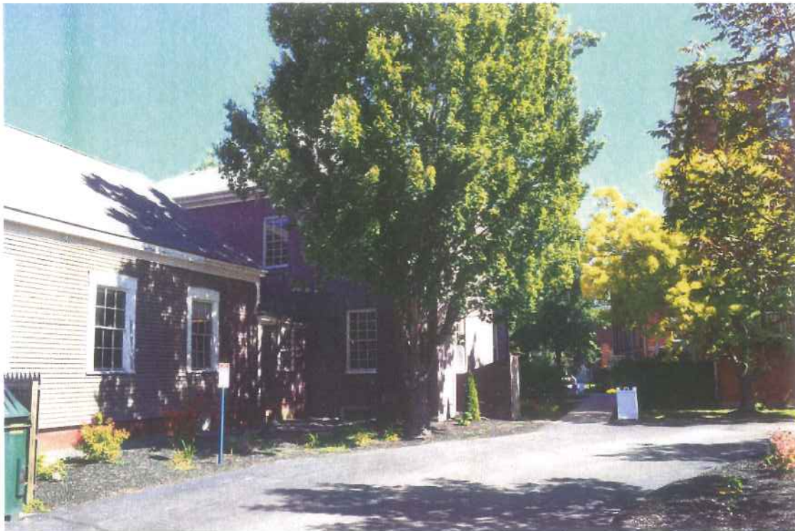
View of Annex from Parking Lot
