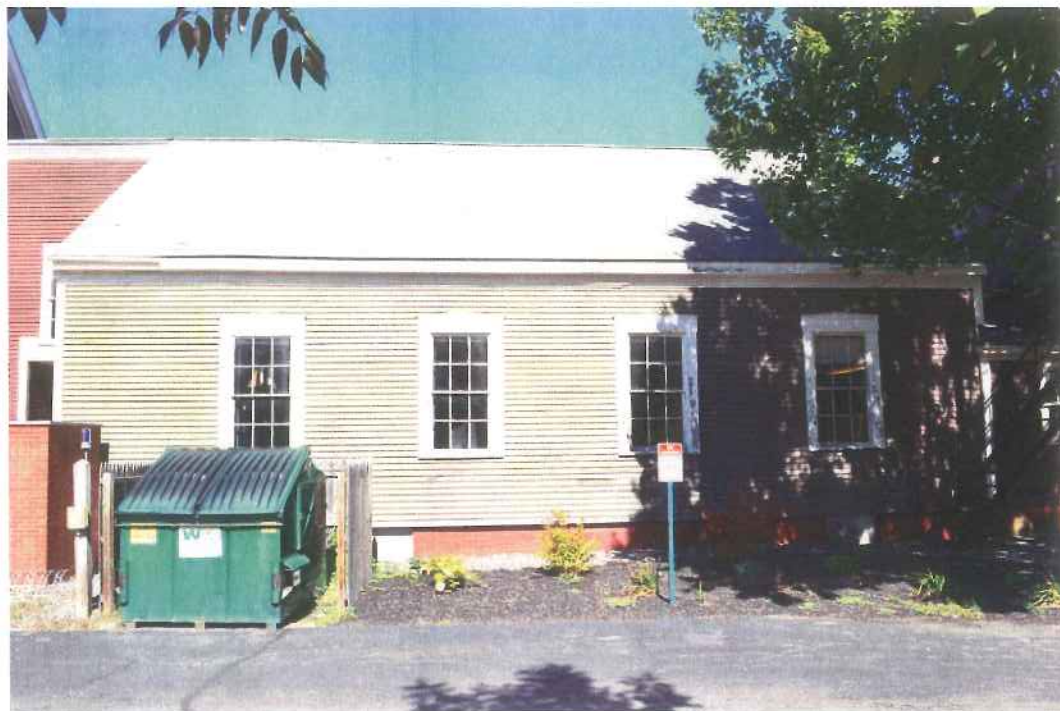
The South Façade of Annex
