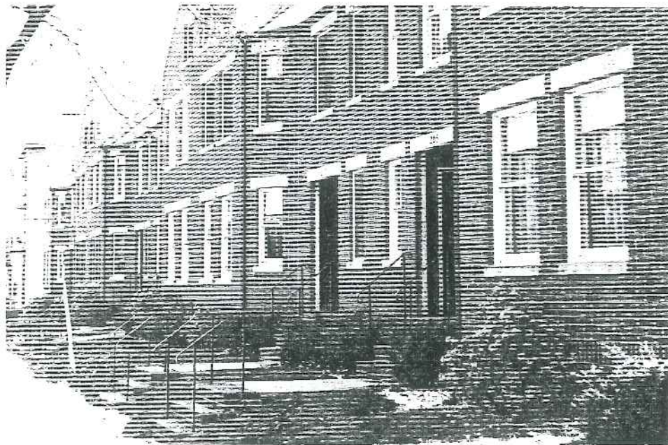
In this condominium townhouse development on Vaughan Street, windows with stone heads and sills, together with recessed entrances, have proportions like those of neighboring historic residences. In addition, the rhythm established by the pattern of the windows and the location of the doors is in common with that of other houses in the district.
