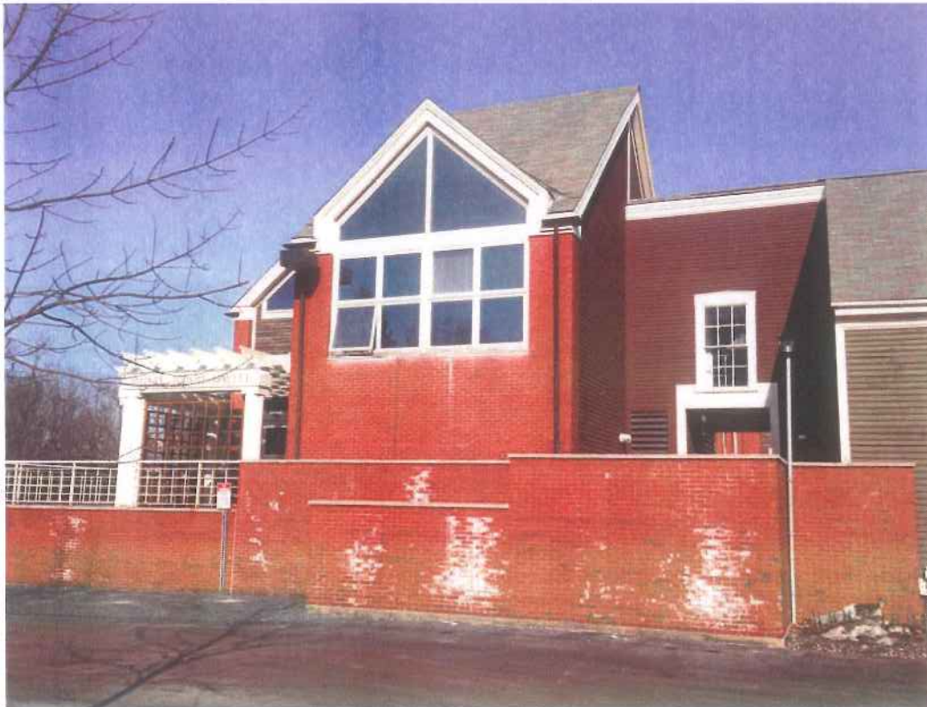
The South Facade of Abplanalp
