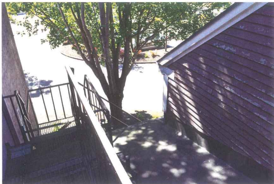
Roof top connection between Alumni and Annex
