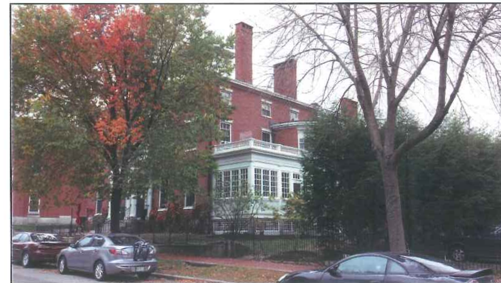
4 SK-4 SITE PICTURE OF MOCK-UP (NOTE : THIS IMAGE SHOWS A 42" TALL PANEL) SCALE: N/A
