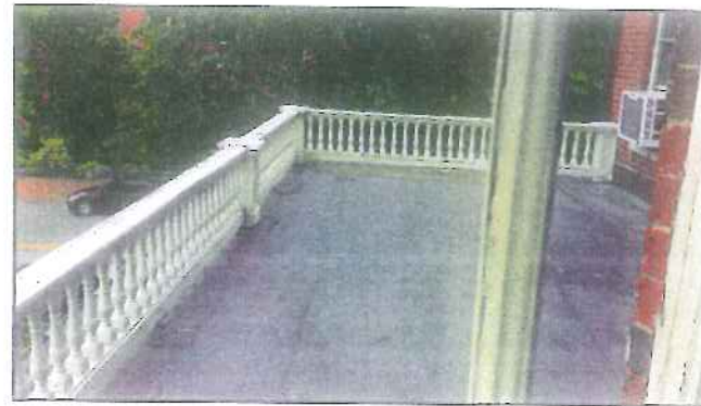
VIEW FROM "OLD PORT" GUEST ROOM
