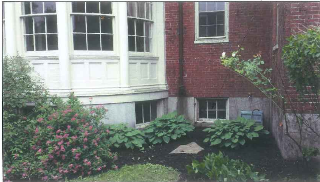
1 SK-2 EXISTING EXTERIOR CONDITIONS SCALE: N/A
