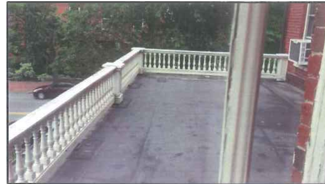
VIEW FROM "OLD PORT" GUEST ROOM
