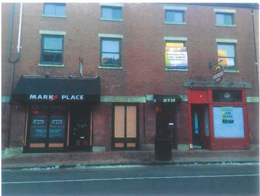
FORE STREET - EXISTING
