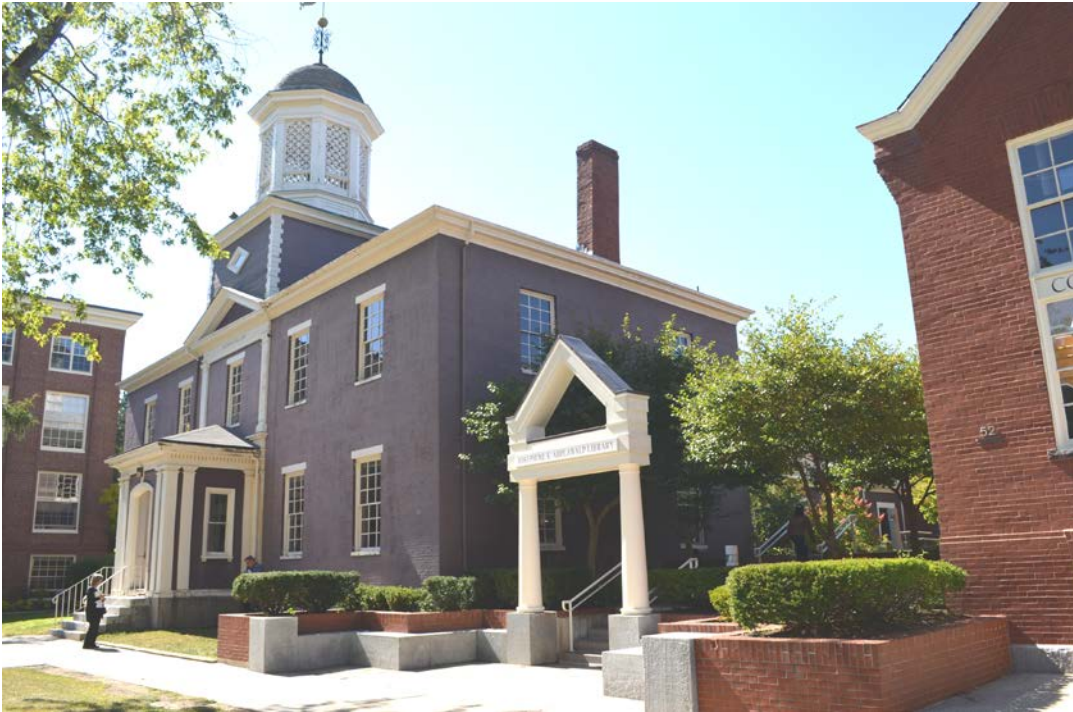
Entrance to Courtyard shared with McArthur
