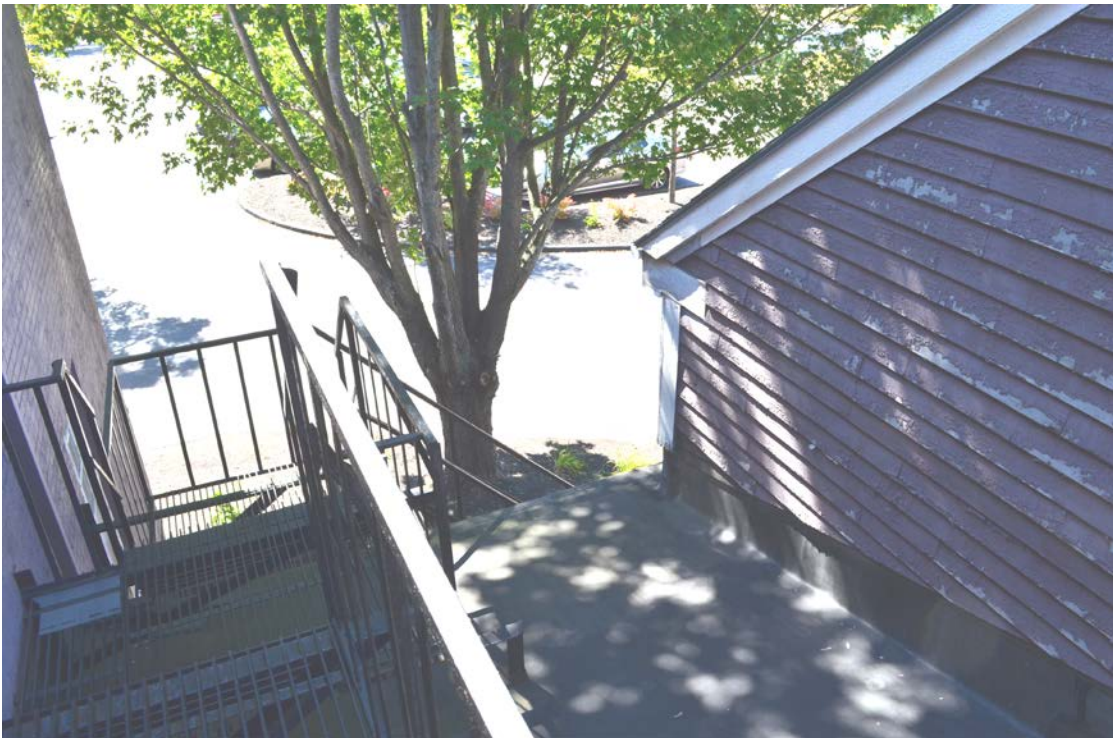
Roof top connection between Alumni and Annex
