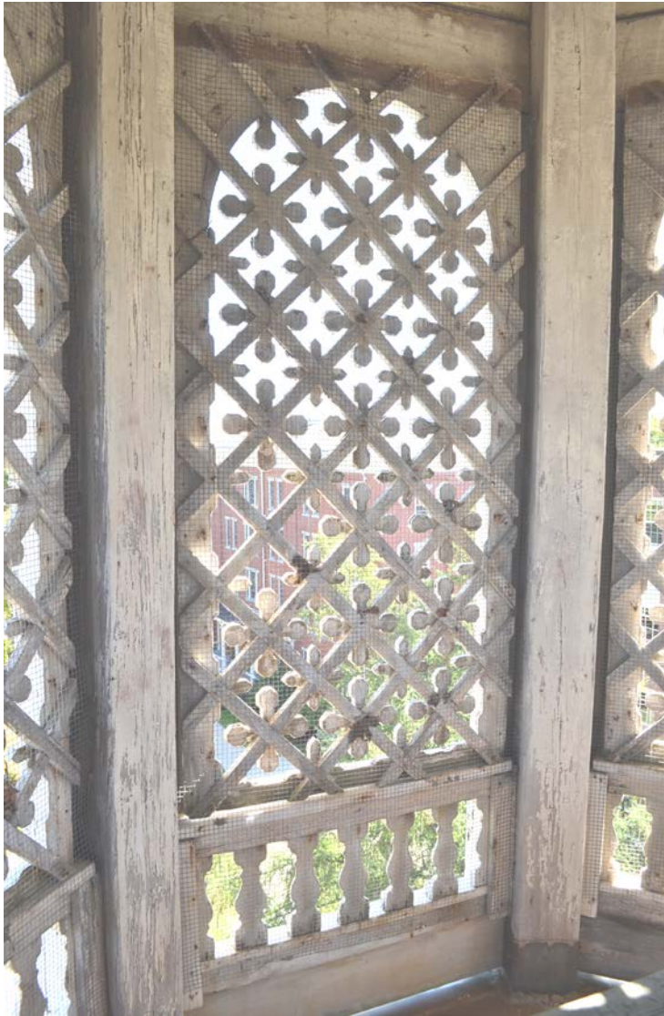
Lattice and Bell in the Cupola
