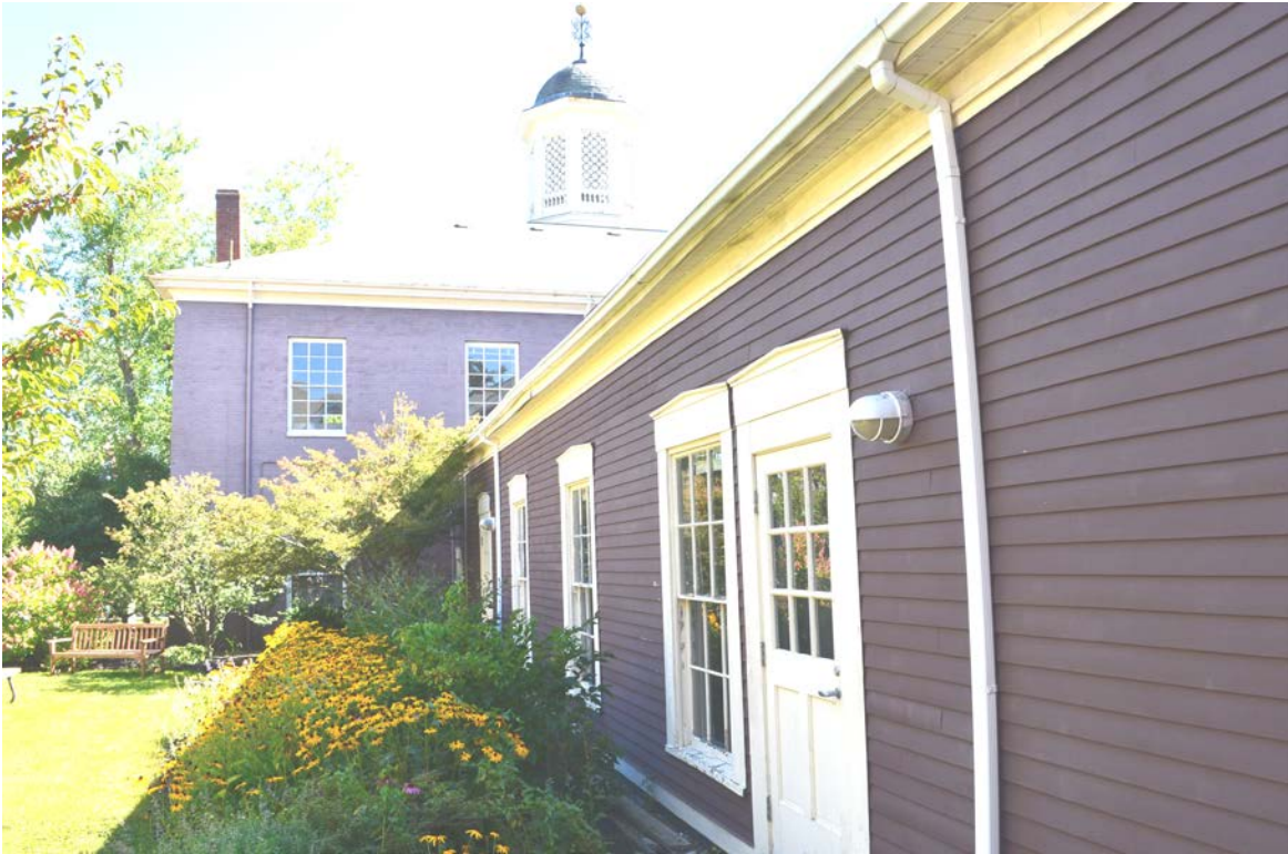
The Annex from the Courtyard
