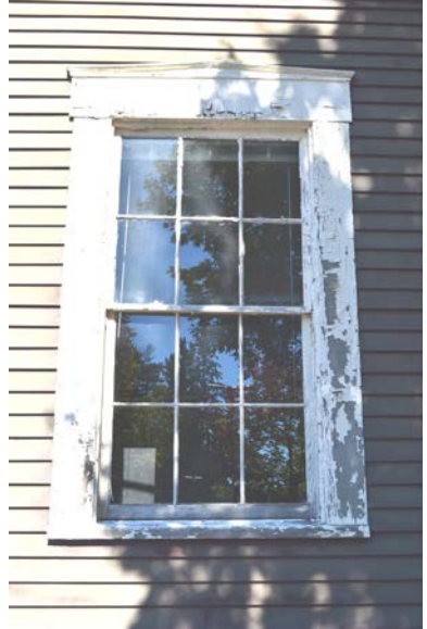
Typical Annex Window
