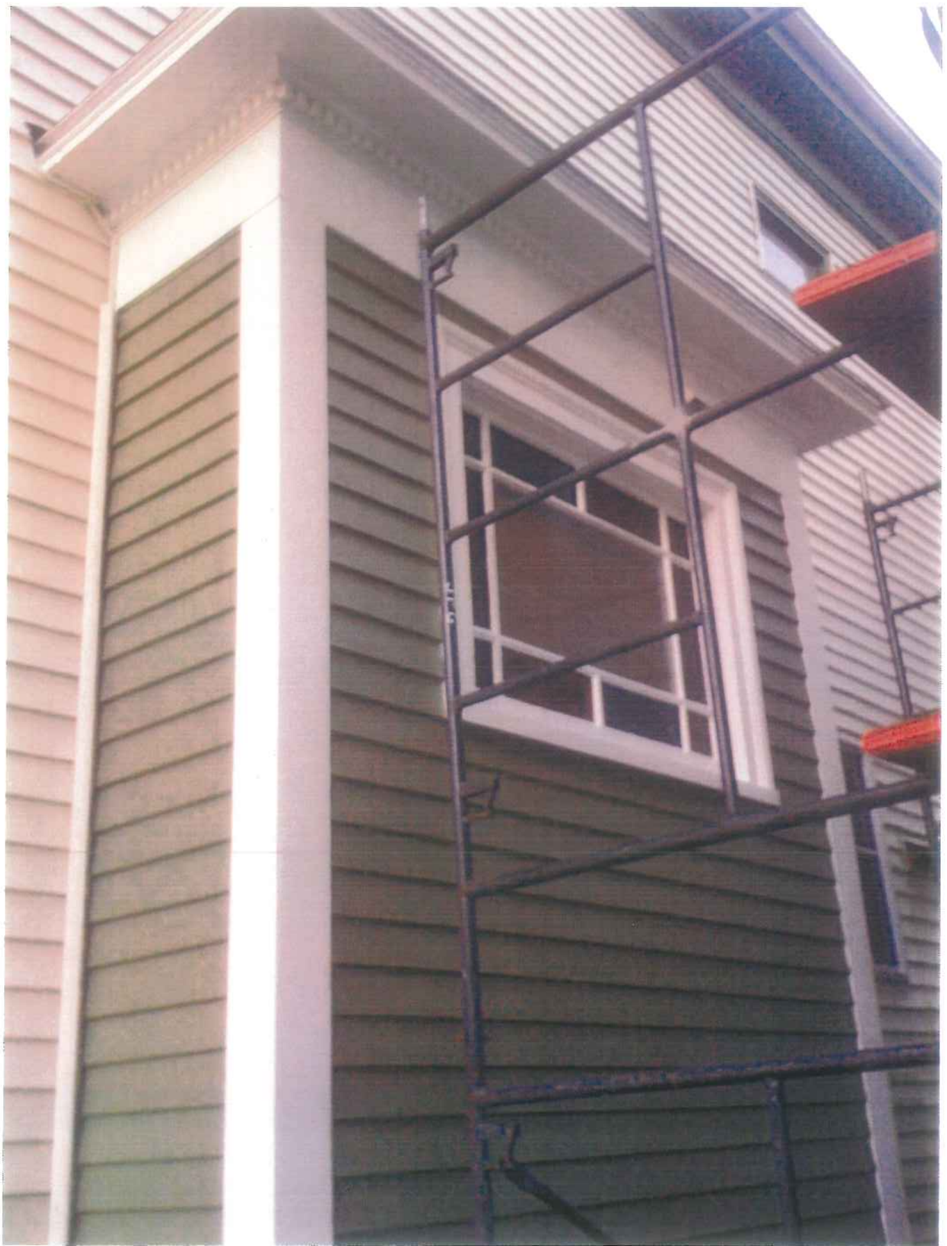
BAY ON EAST FACADE
