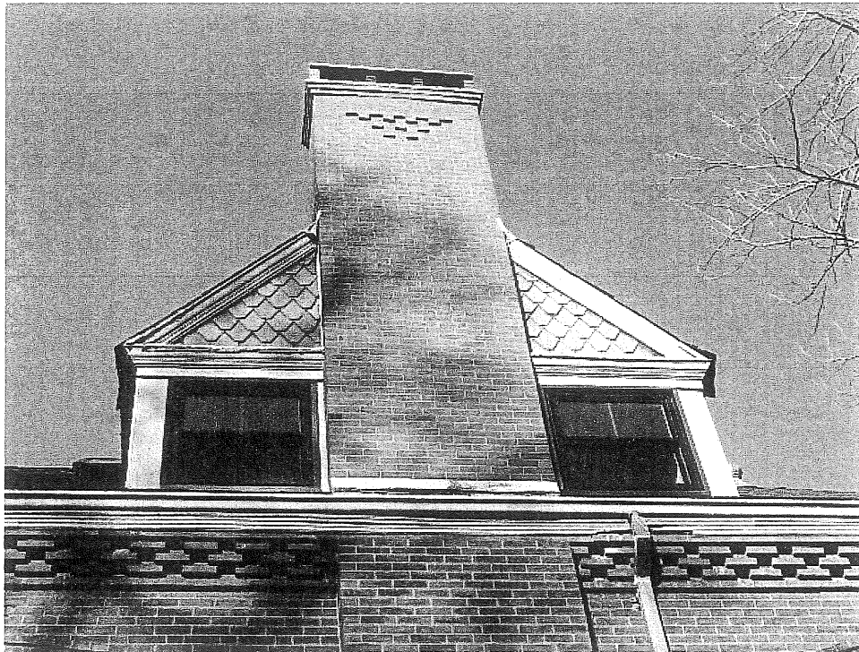
Existing South facing Bisected Dormer
