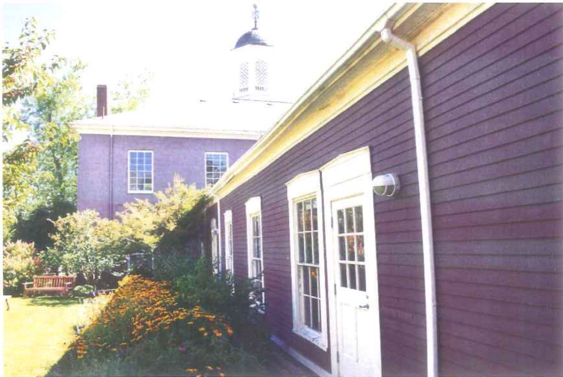
The Annex from the Courtyard
