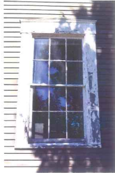
Typical Annex Window
