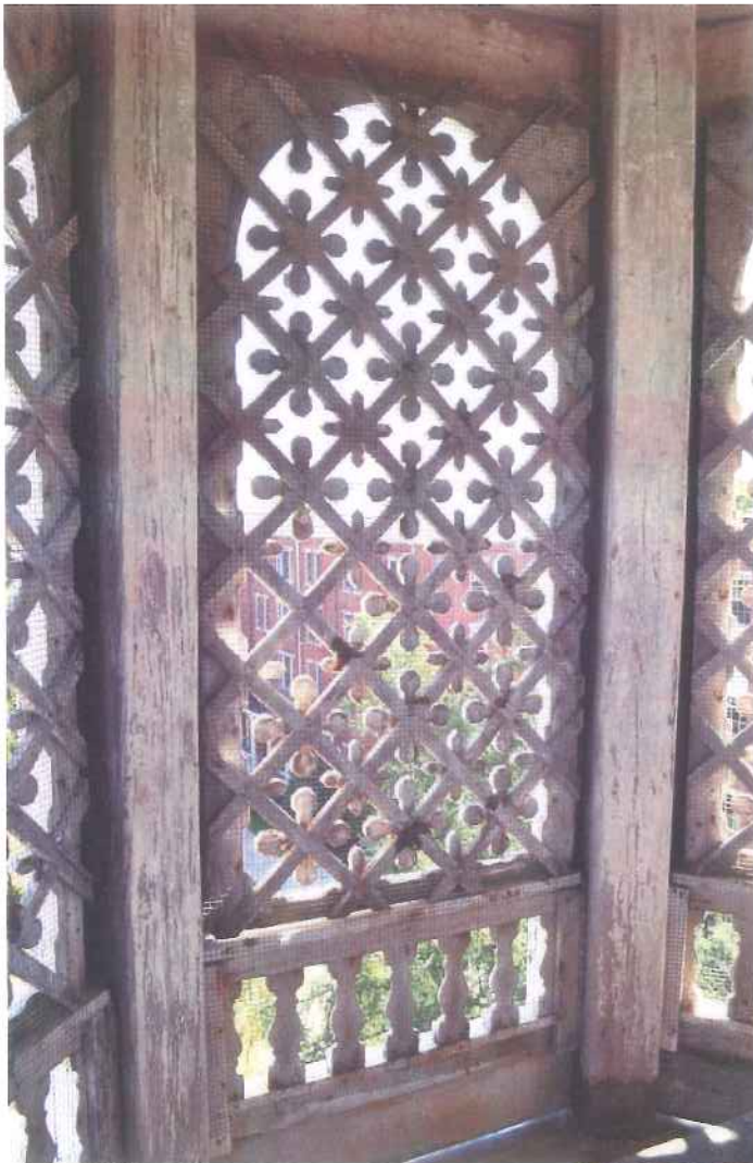
Lattice and Bell in the Cupola
