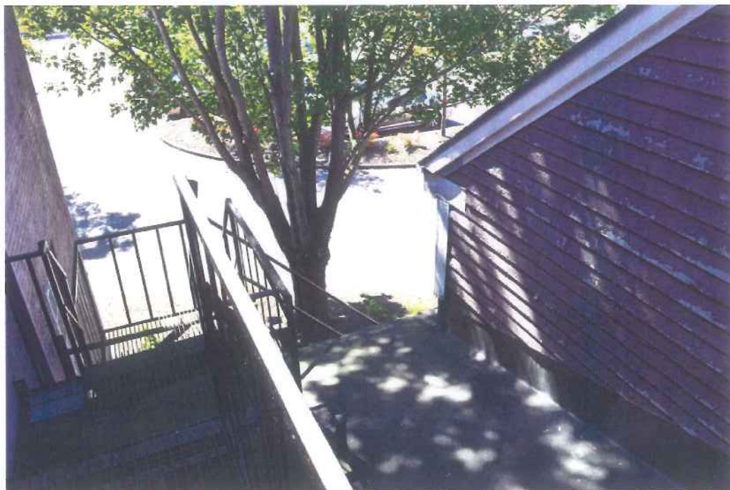
Roof top connection between Alumni and Annex
