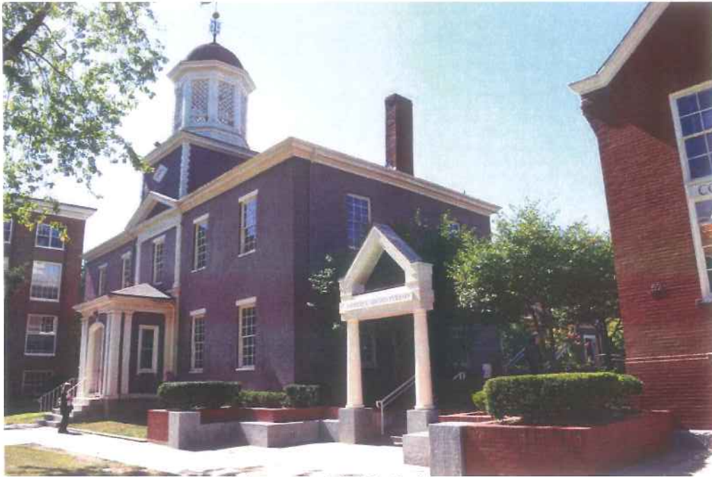
Entrance to Courtyard shared with McArthur
