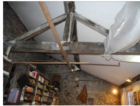
Queen Rod Truss in Building 6B (left); King Post Truss in Building 14 (right)
