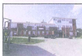
Building 30: Office Construction Date: 1950
