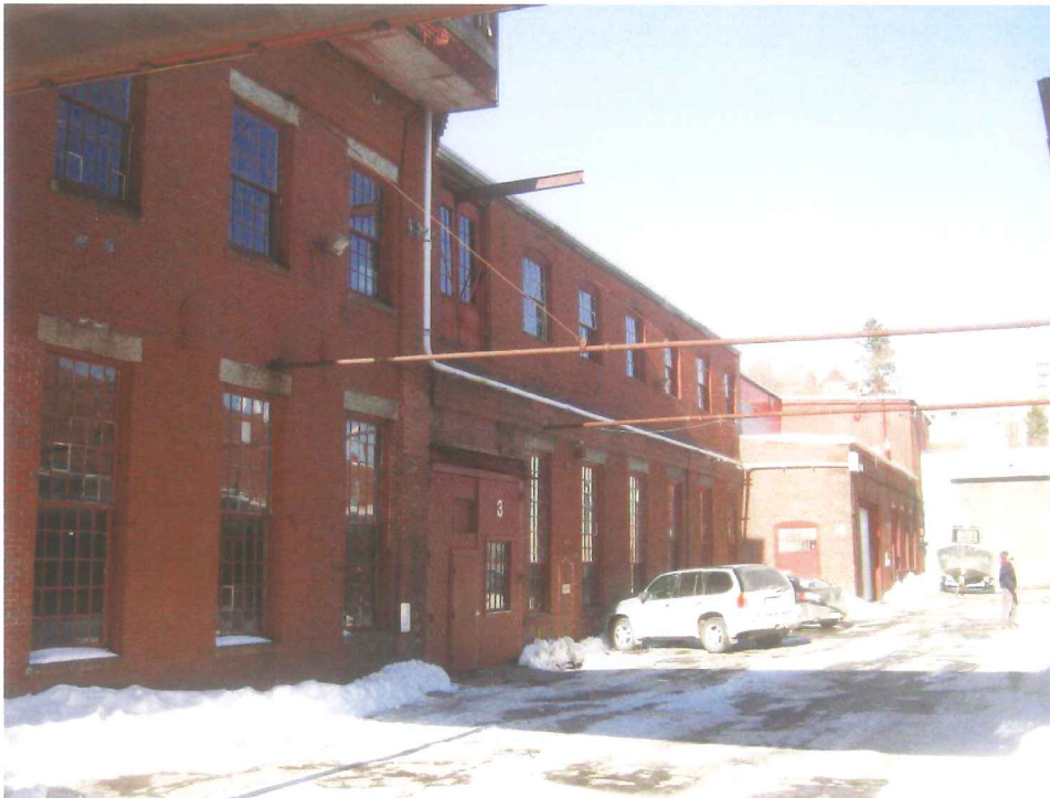
Photo 3-1: Exterior view of Building 3
