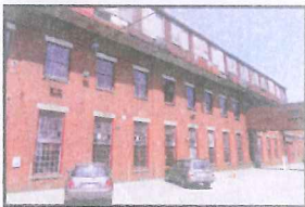
Building 2: Machine Shop Construction Date: c. 1847 Alterations: c. 1905: Addition of office dormers to third floor
