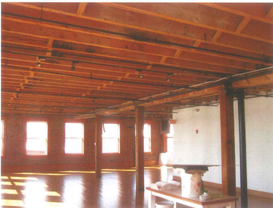
Photo 6A-2: General view of center bearing line of Building 6A at second floor level.
