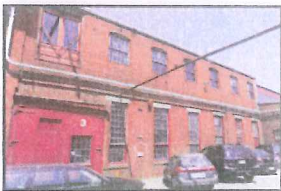
Building 3: Machine Shop Construction Date: c. 1847 Alterations: c. 1895: Addition of second floor
