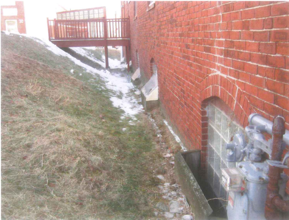
Photo 11-4: Window wells and embankment at north wall.
