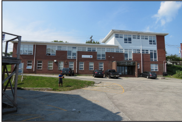
Building 30: Office Construction Date: 1950
