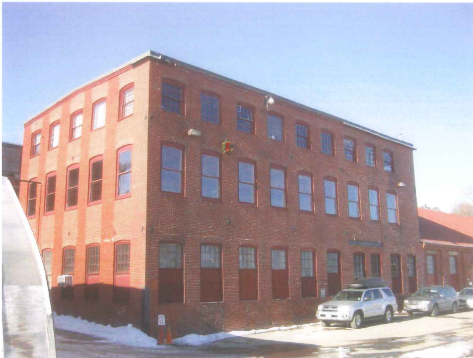
Photo 6A-1: Building 6A exterior view.
