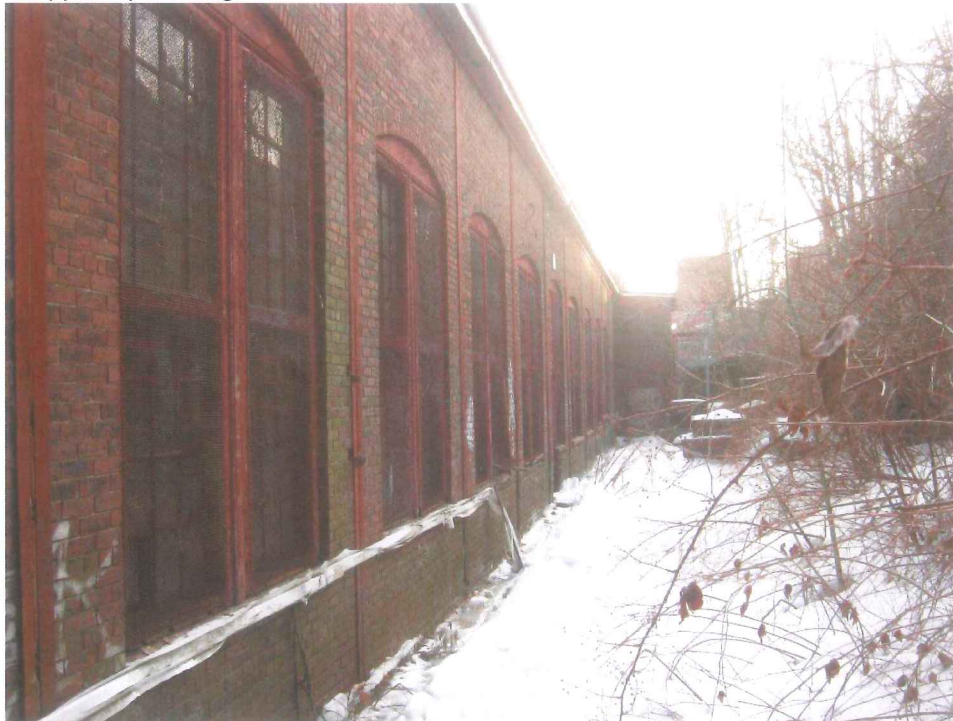
Photo 4-2: Exterior of Building 4, North Side.
