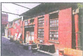
Building 15 & 16: Boiler House & Brass Foundry Construction Date: 1858-64; 1984-71 Alterations: c. 1980: Loss of original smokestack
