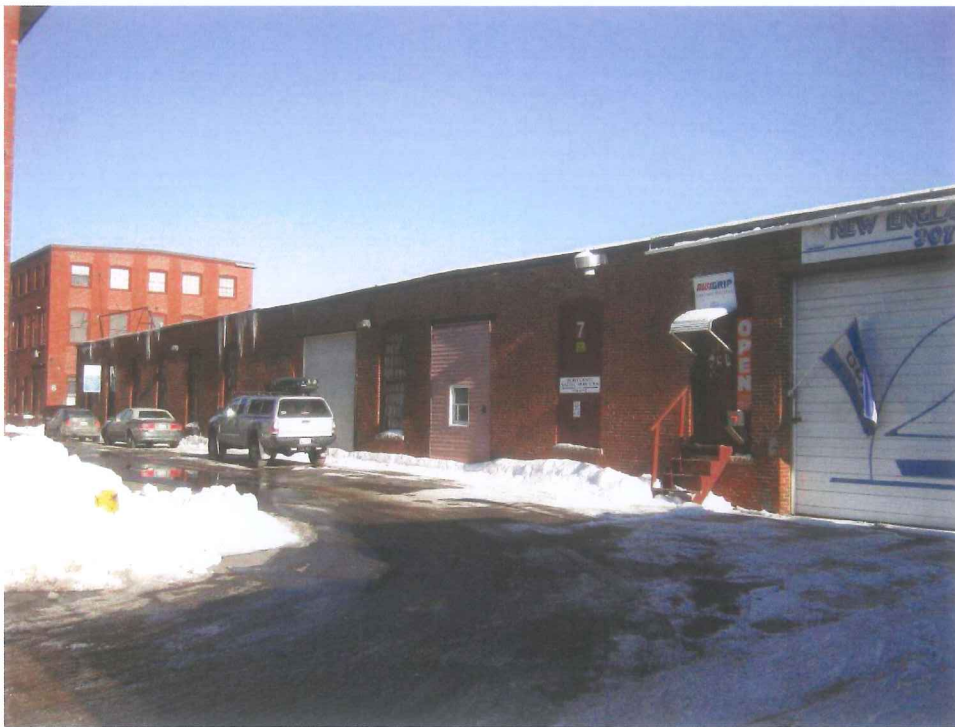
Photo 7-2: North elevation of Building 7.
