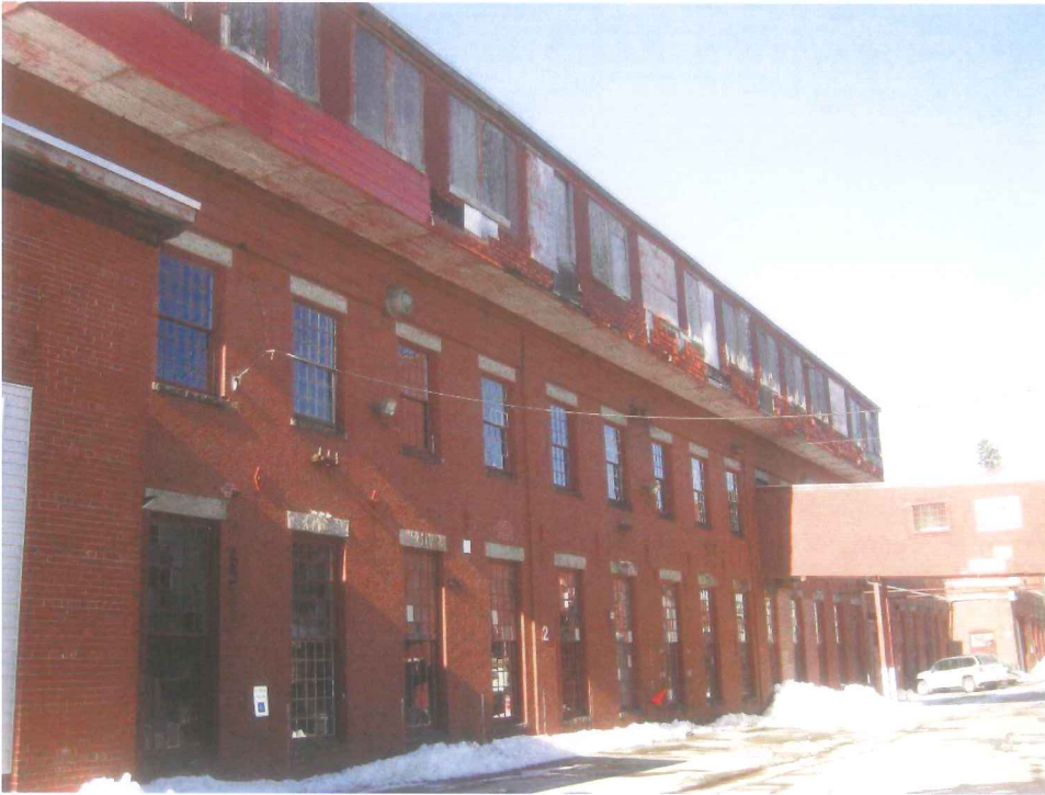
Photo 2-1: Building 2 exterior south elevation.
