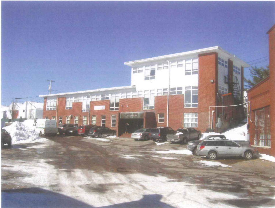
Photo 30-1: Southwest elevation of building 30.
