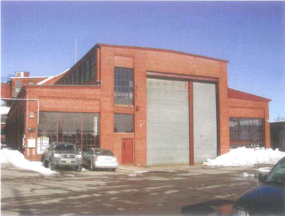
Photo 1-1: General View, Building 1
