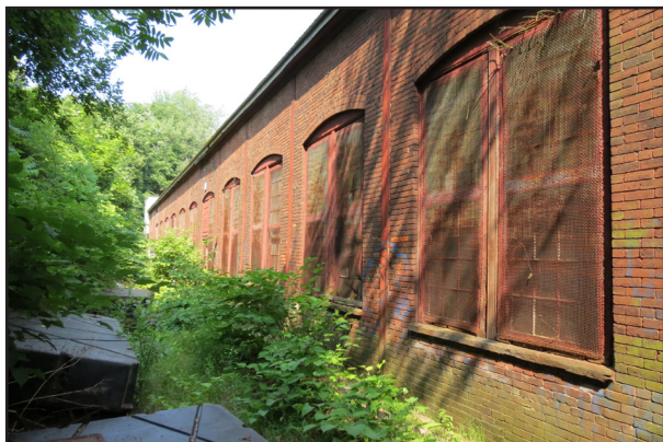
Building 4: Foundry and Acetylene House Construction Date: 1895; 1904-09
