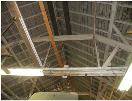
Queen Rod Truss in Building 6B (left); King Post Truss in Building 14 (right)
