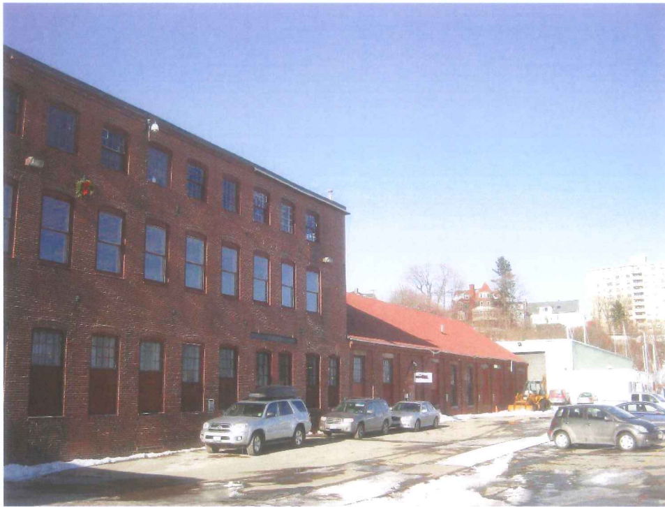
Photo 6B-1: Buildings 6A (left) and 6B (right).
