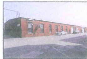
Building 7: Car Shop Construction Date: c. 1873 Alterations: c. 1904: Addition of lumber storage building
