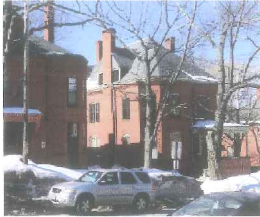
View from State Street
