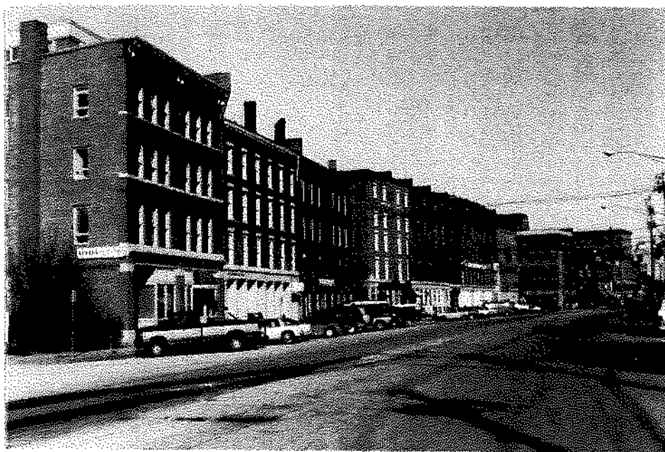
North side of Commercial Street.
