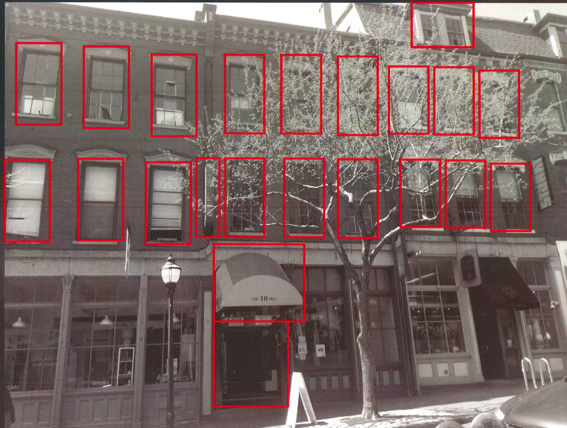
10 Exchange Street – Exchange Street Proposed Demo/Upgrade
