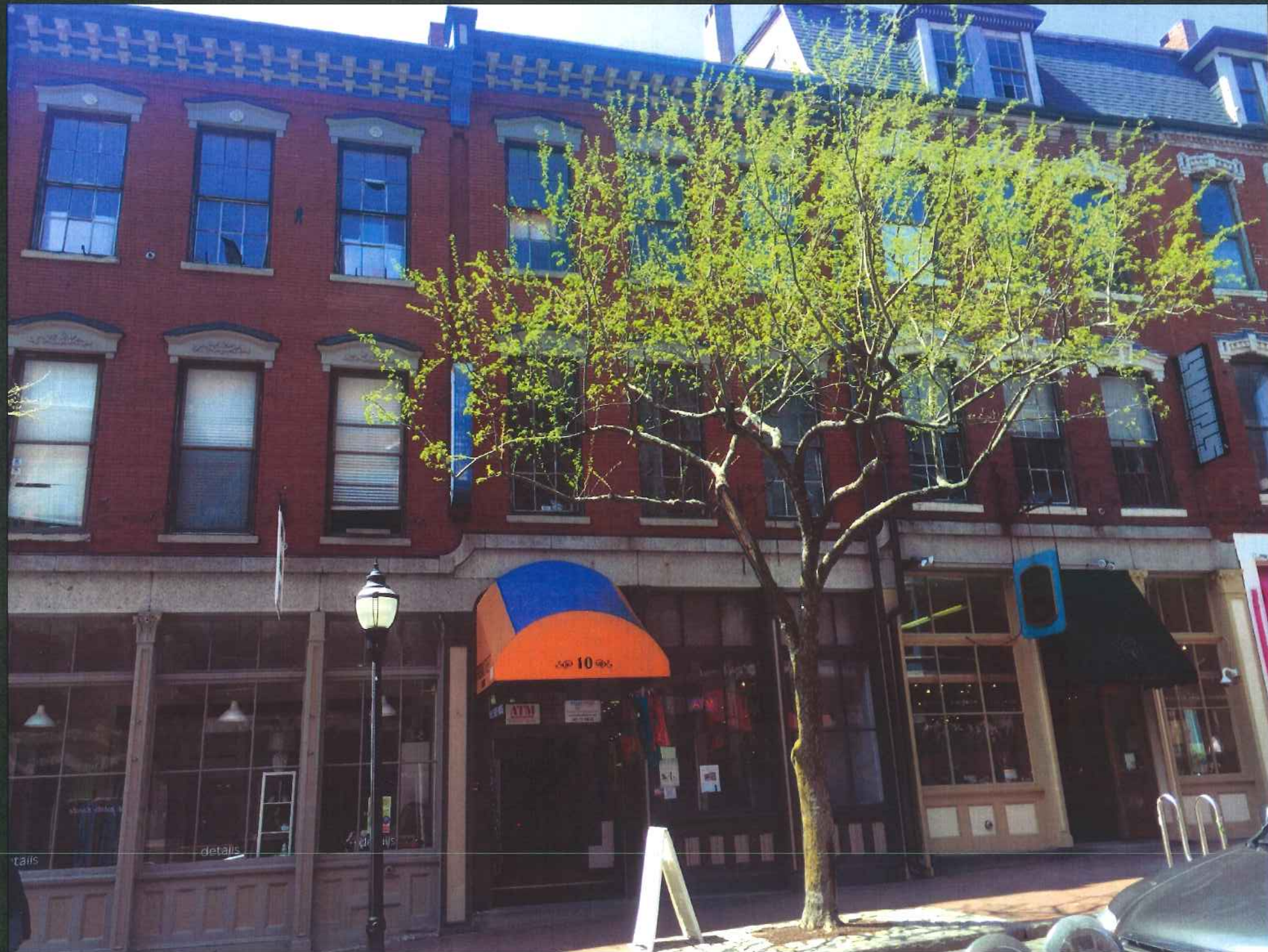
10 Exchange Street – Exchange Street Existing Facade
