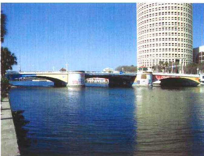
Kennedy Blvd. Bridge, constructed 1913
