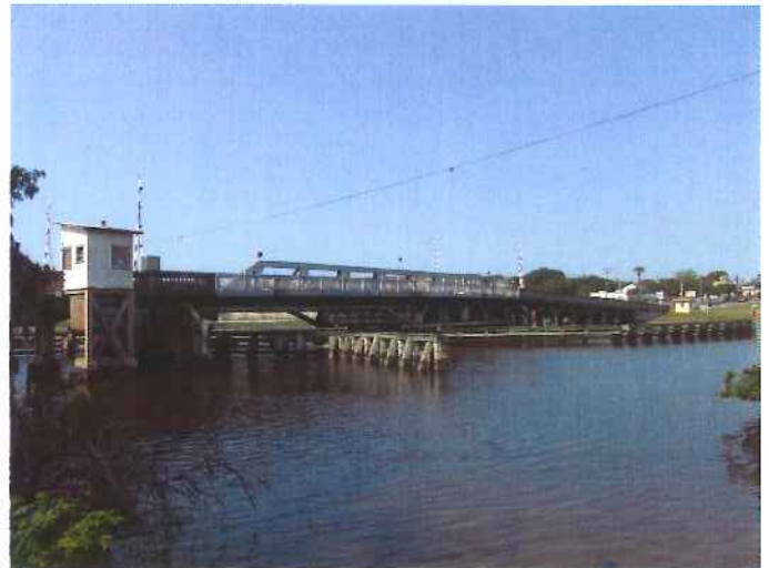
Columbus Drive Bridge, constructed 1927
