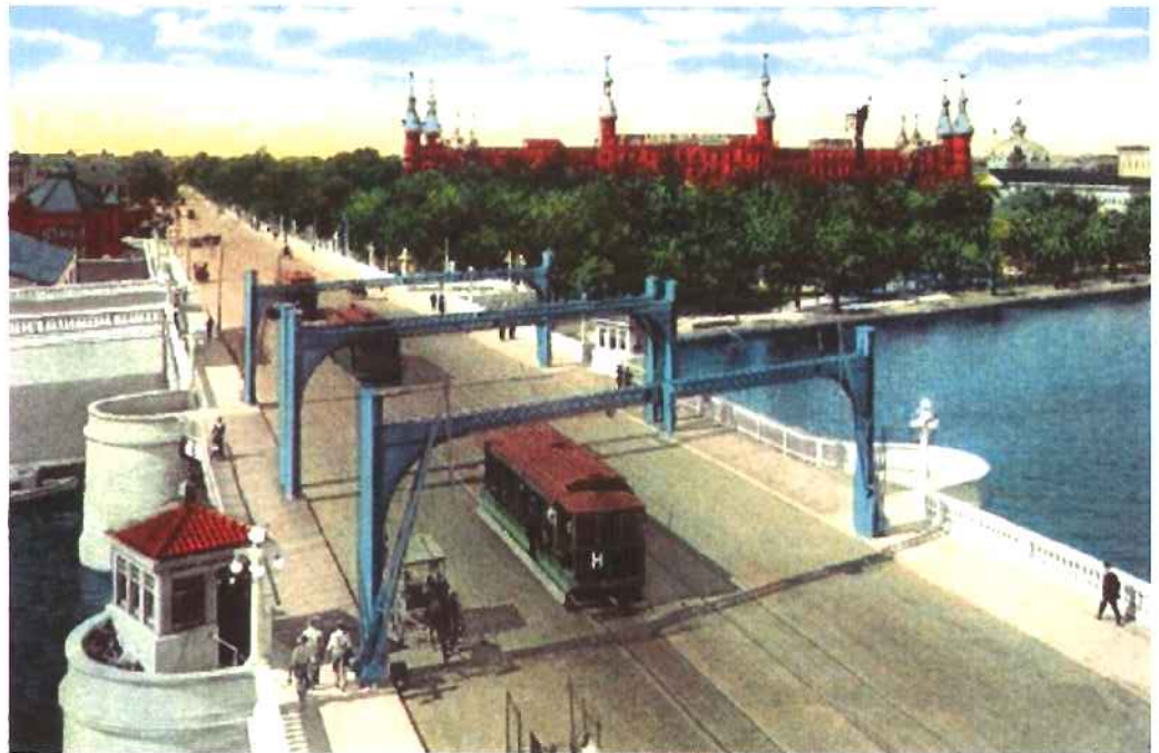
Lafayette Street Bridge, date unknown
