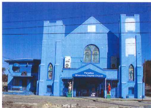
Paradise Missionary Baptist Church 1112 Scott St., constructed 1924
