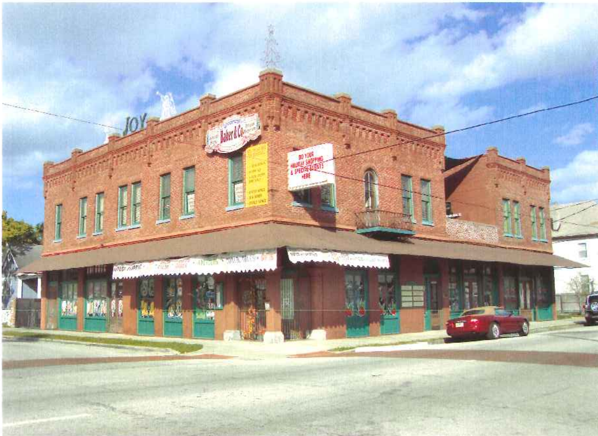
2502 North Howard Ave., constructed 1903
