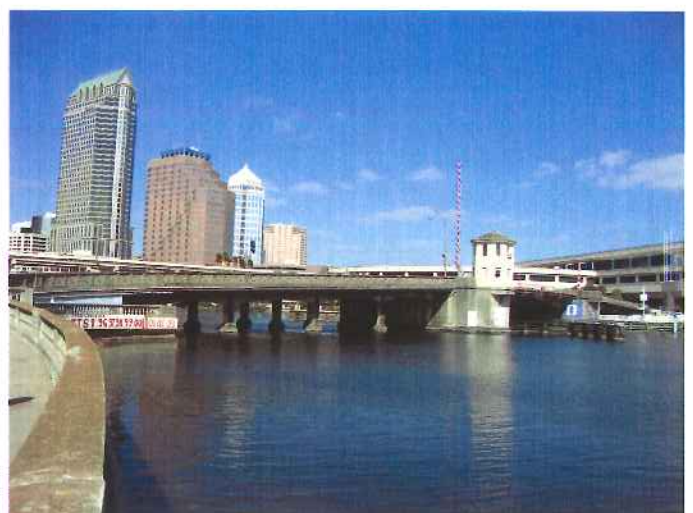
Platt Street Bridge, constructed 1926
