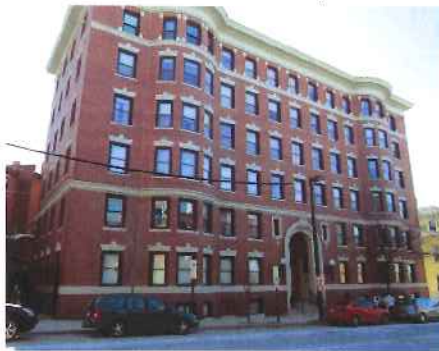
Bay projections, Base/Middle/Top, Delineation of floors, Lintels, Recessed entry, Overhang cornice
