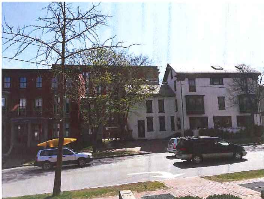
VIEW LOOKING EAST FROM STATE STREET
