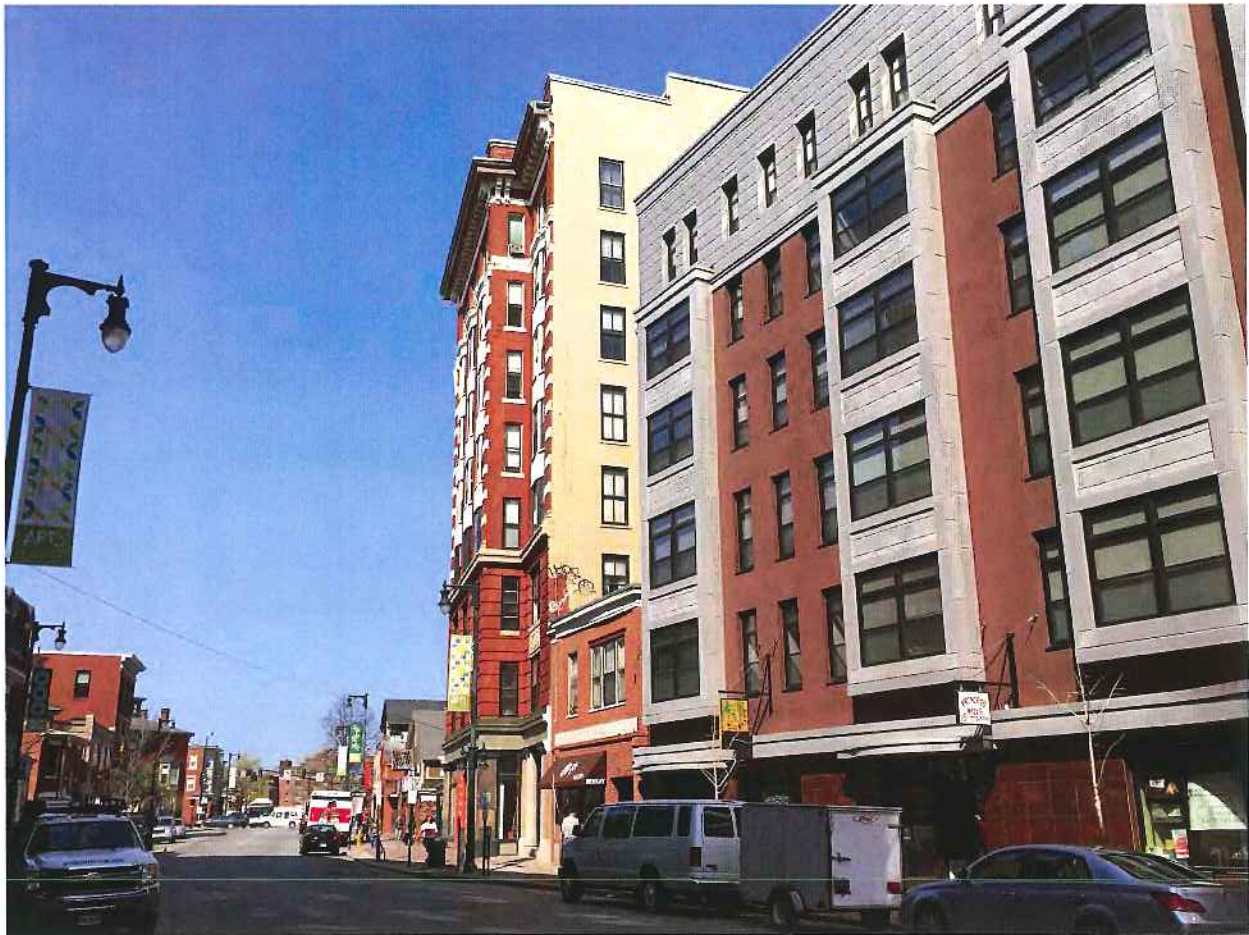
VIEW LOOKING EAST ON CONGRESS ST
