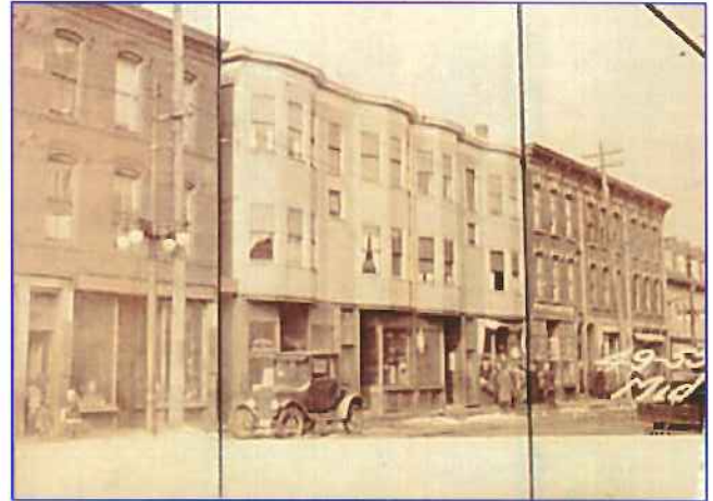
Reflecting the neighborhood's multicultural nature and tradition of living above one's place of business, this 3-family building on Middle Street with store on the ground floor was owned by Hyman Finklestein in 1924. The flanking brick buildings remain.
