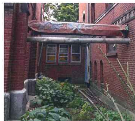
West facade of 'Connector' piece facing parking
