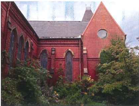
South facade facing the Courtyard
