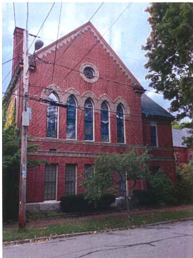
East facade facing Thomas Street
