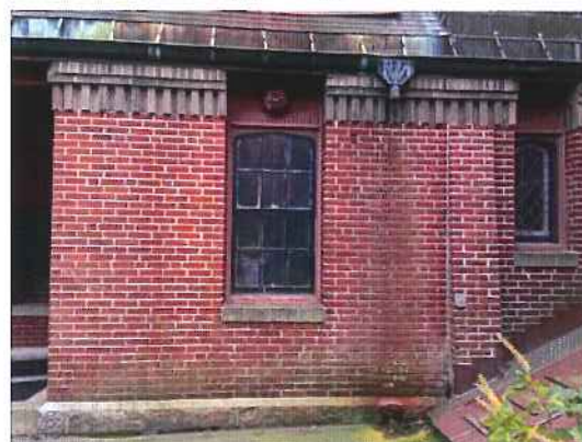
North facade facing Courtyard - featuring entrance portico and illustrating current condition of brick and limestone detailing
