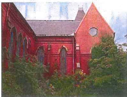
South facade facing the Courtyard
