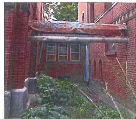
West facade of 'Connector' piece facing parking
