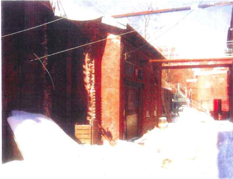
Photo 16-1: Exterior view of blacksmith shop/Building 16.
