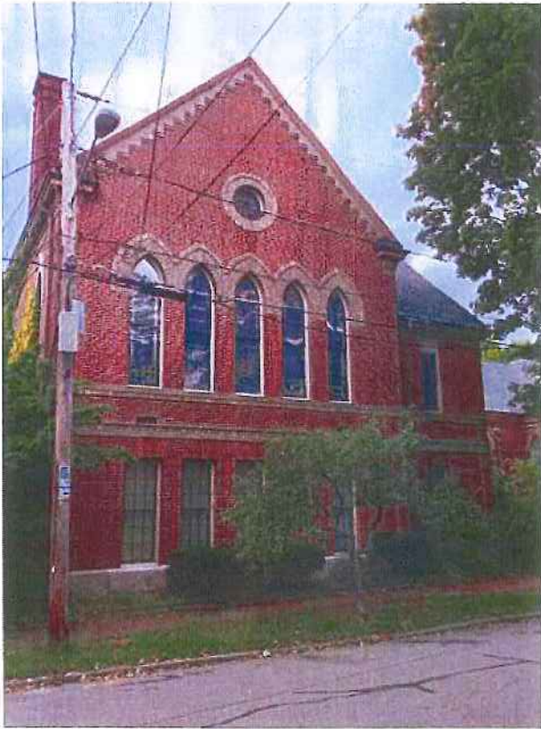
East facade facing Thomas Street
