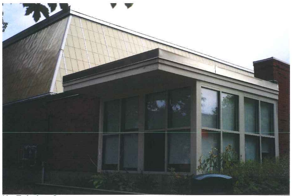
H - Existing Gym
