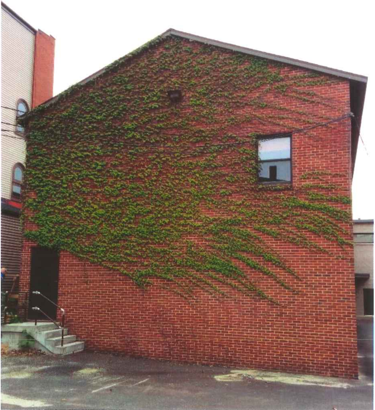
Rear (West) Façade
