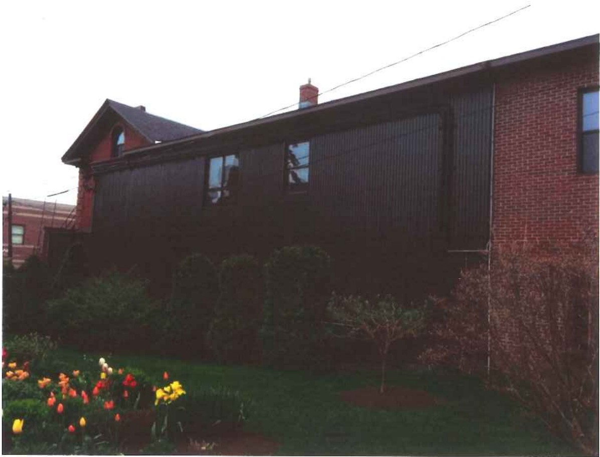
Façade – North Elevation
