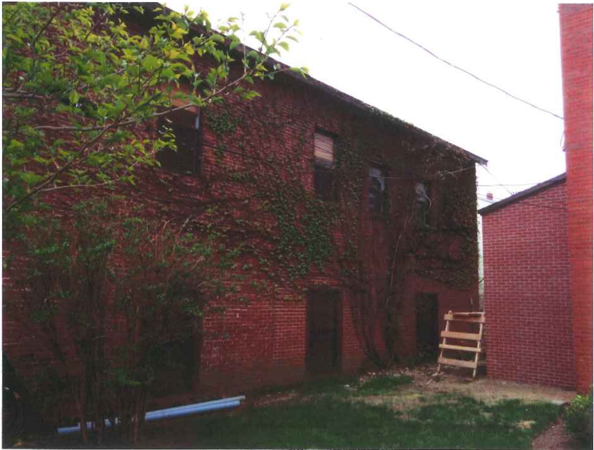
Façade – North Elevation
