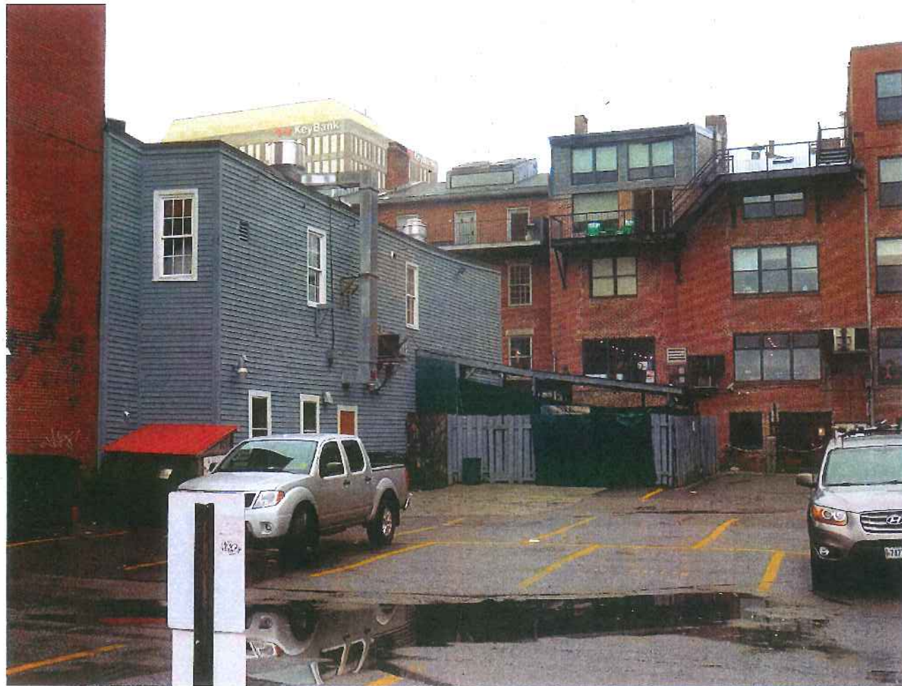
3a Existing view from Commerical Street NTS
