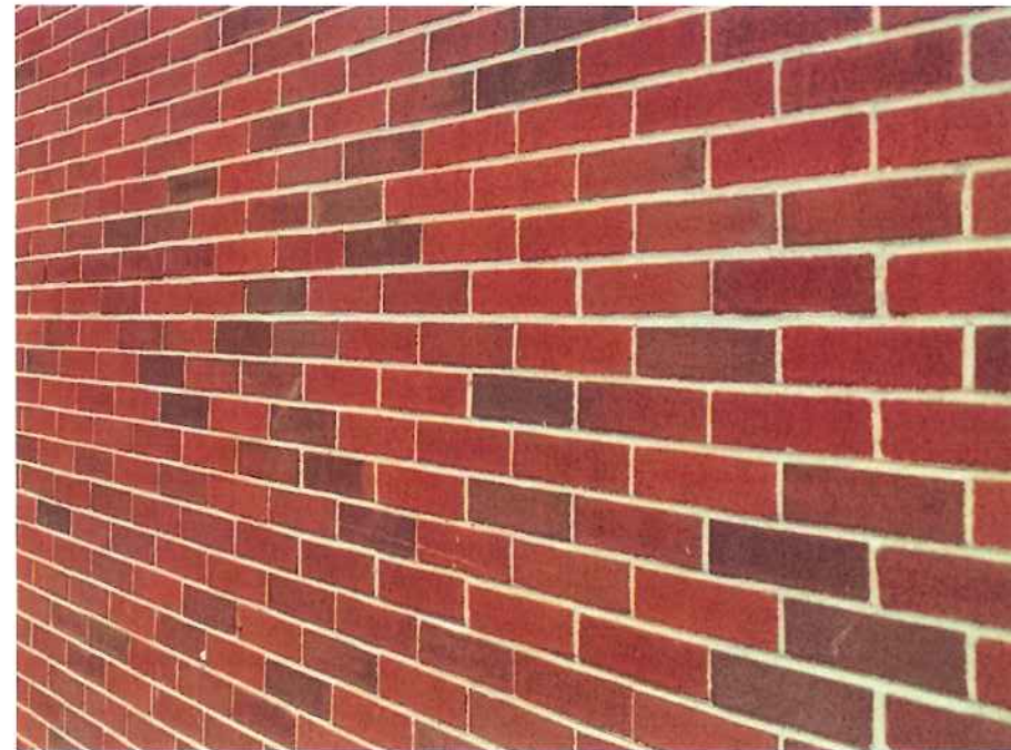
TYPICAL BRICK - 12" NORMAN BRICK TO MATCH EXISTING
