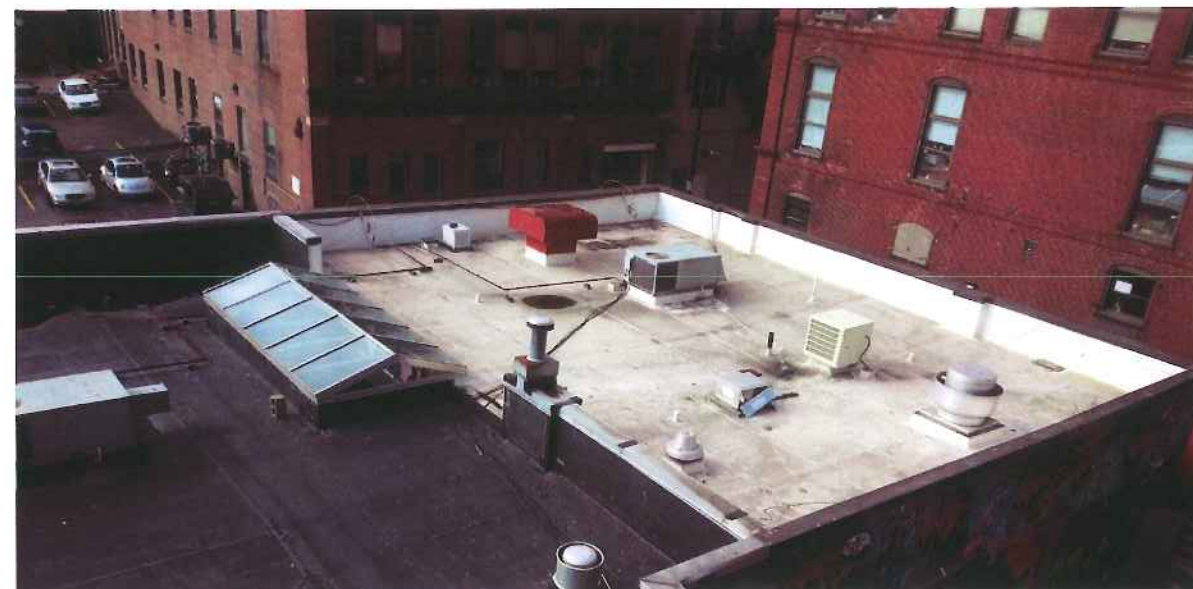
Asylum / Free Street Live - Event Space Renovation November 25th, 2015
