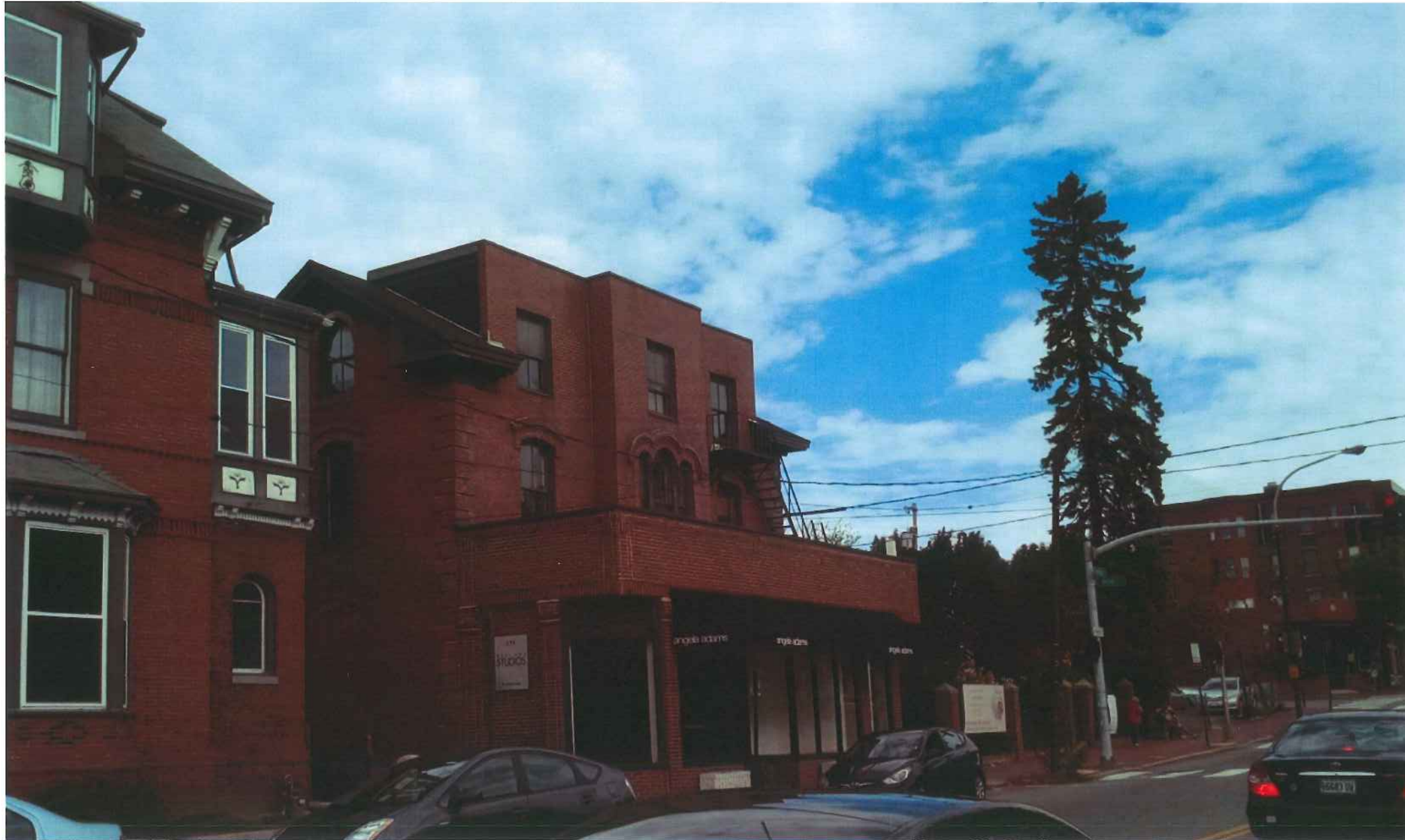
Existing view of front façade
