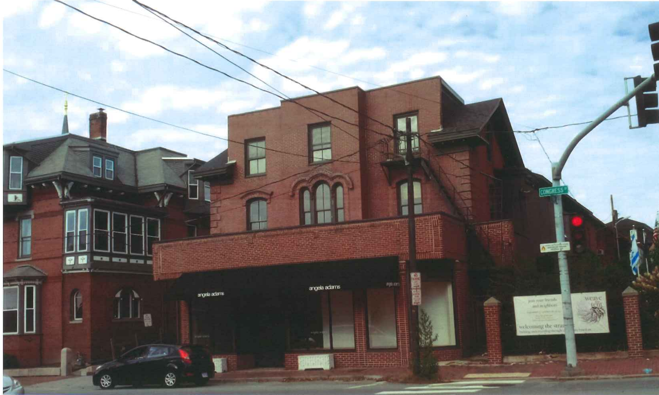
Existing view of front façade
