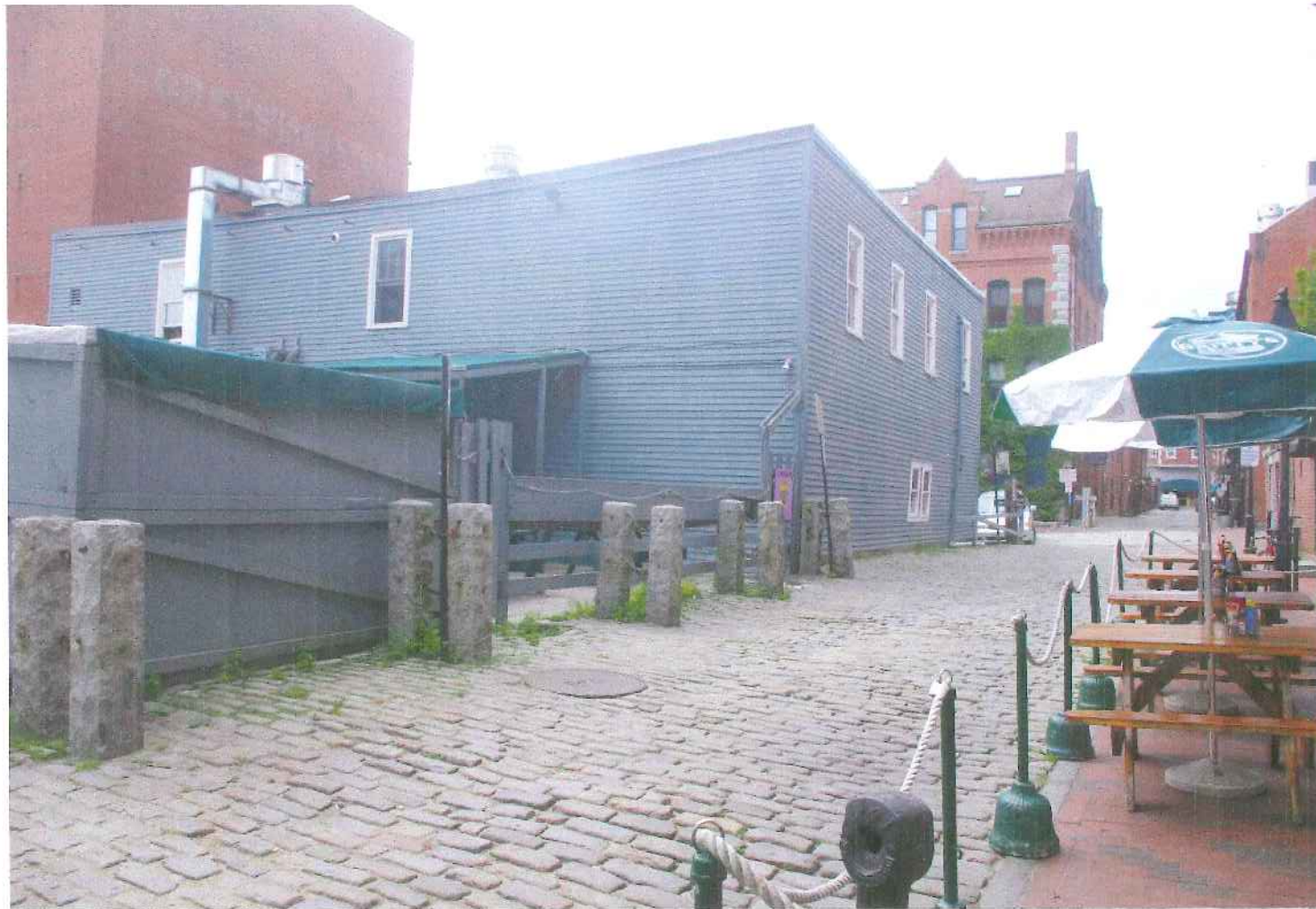
a Existing view from Wharf Street, looking South NTS
