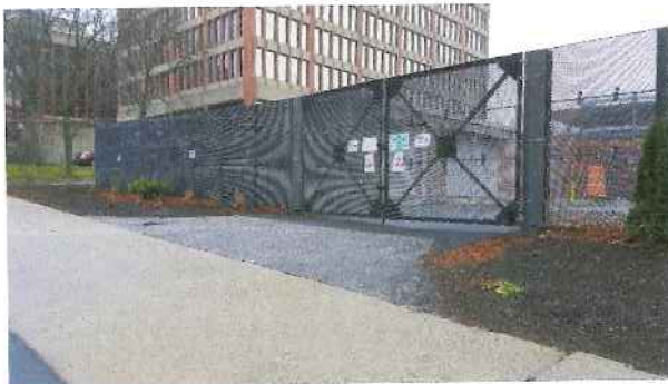
Behind Hyatt Place: Steel diamond grid
