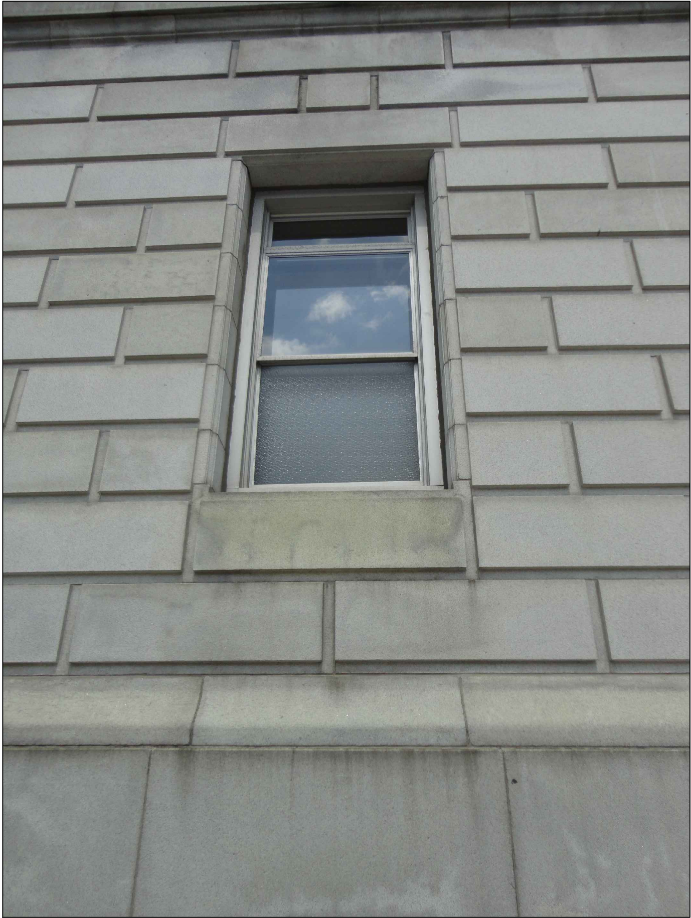
FIRST FLOOR WINDOW
