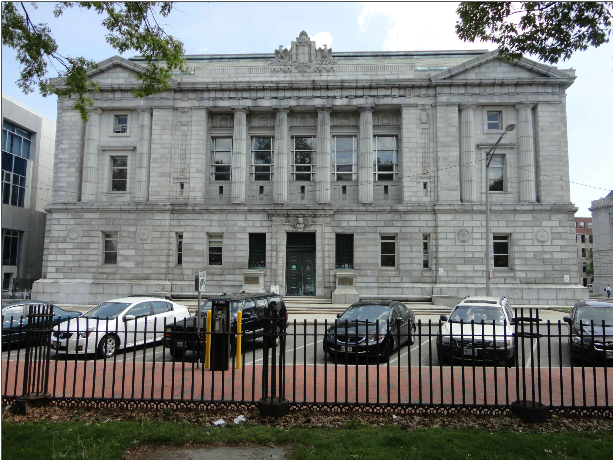
FEDERAL STREET FACADE
