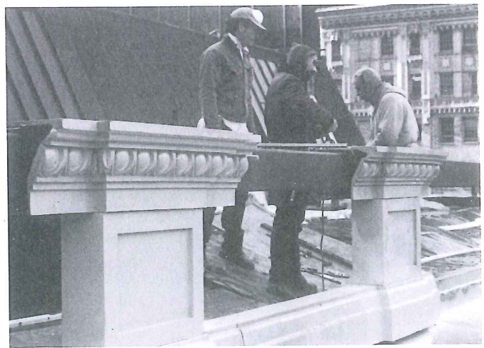
Illus. 18. Substitute materials must be properly installed to allow for expansion, contraction, and structural security. The new balustrade (a polymer concrete modified with glass fibers) at Carnegie Hall, New York City, was installed with steel structural supports to allow window-washing equipment to be suspended securely. In addition, the formulation of this predominantly epoxy material allowed for the natural expansion and contraction within the predesigned joints. Photo: Courtesy of MJM Studios.
