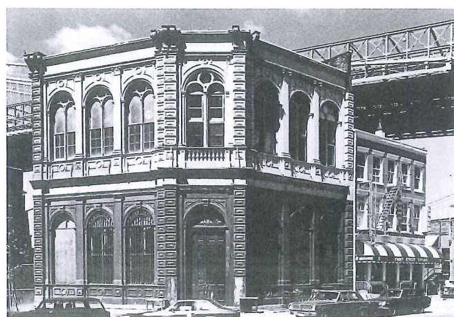
Illus. 4. The 19th-century also produced a variety of metal products used in imitation of other materials. In this case, the entire exterior of the Long Island Safety Deposit Company is cast-iron representing stone. Photo: Becket Logan, Friends of Cast Iron Architecture.
