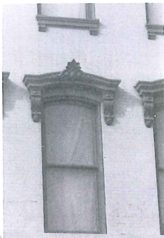
Illus. 5. The four historic examples of various window hoods shown are: (a) stone; (b) cast stone; (c) cast-iron; and (d) sheet metal. The criteria for selecting substitute materials today (availability, quality, delivery dates, cost) are not much different from the past. Photo: Sharon C. Park, AIA.
