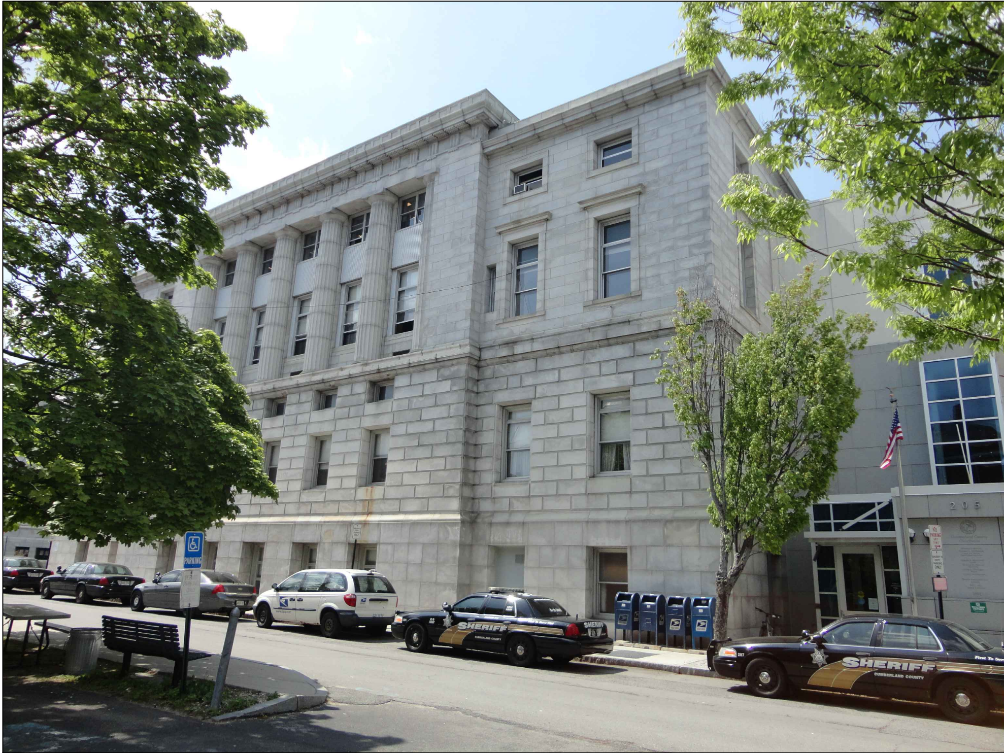
NEWBURY STREET @ CONNECTION TO NEW ADDITION
