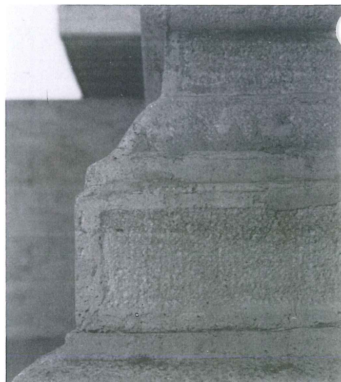
Illus. 15. Poor quality workmanship can be avoided. In this example, the crudely cast concrete entrance pier (shown) did not match the visual qualities of the remaining historic sandstone (not shown). The aggregate is too large and exposed; the casting is not crisp; the banded tooling edges are not articulated; and the color is too pale. Photo: Sharon C. Park, AIA.
