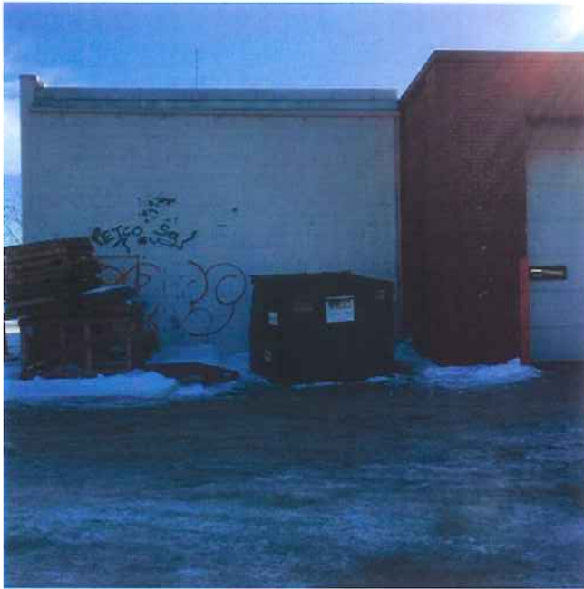
Newer addition at back of building with cmu walls
