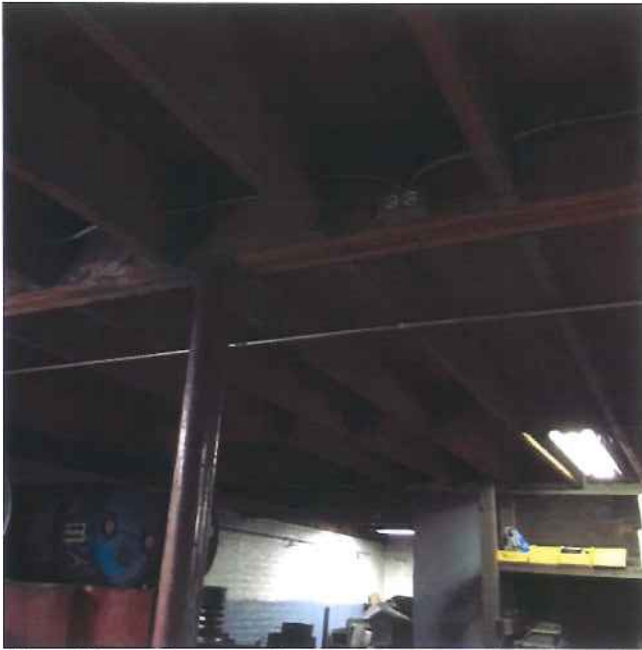
Wood framed mezzanine at newer warehouse addition
