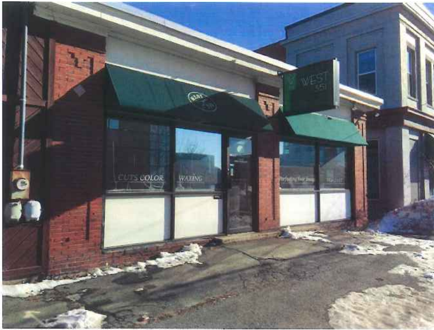
Front elevation view of 351 Forest Avenue
