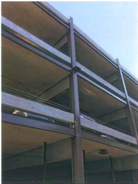
Image-03 West (Hyatt Place) facade showing garage after brick is removed, steel refurbished and galvanized automobile guard added.
